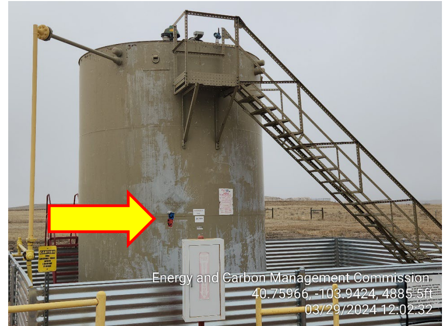
Photo 12 – Maintenance Tank – NFPA and Content Labels
