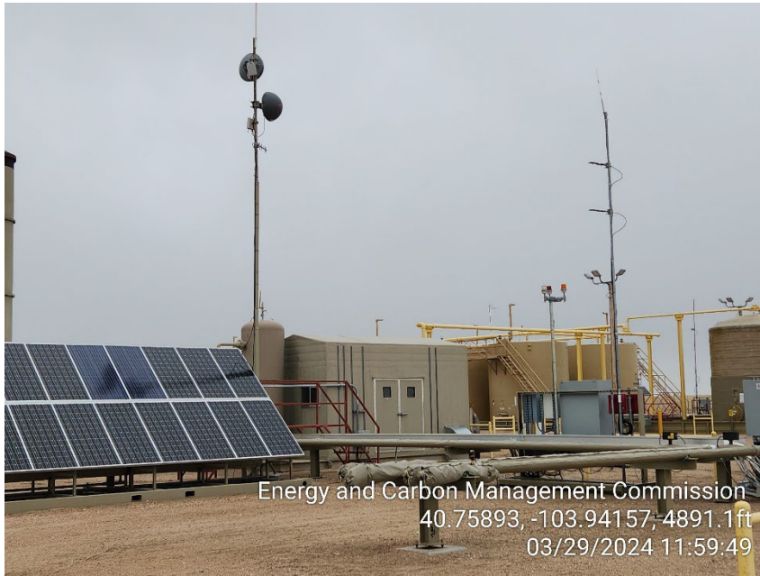
Photo 3 – Instrumental Air Unit and Solar Panels
