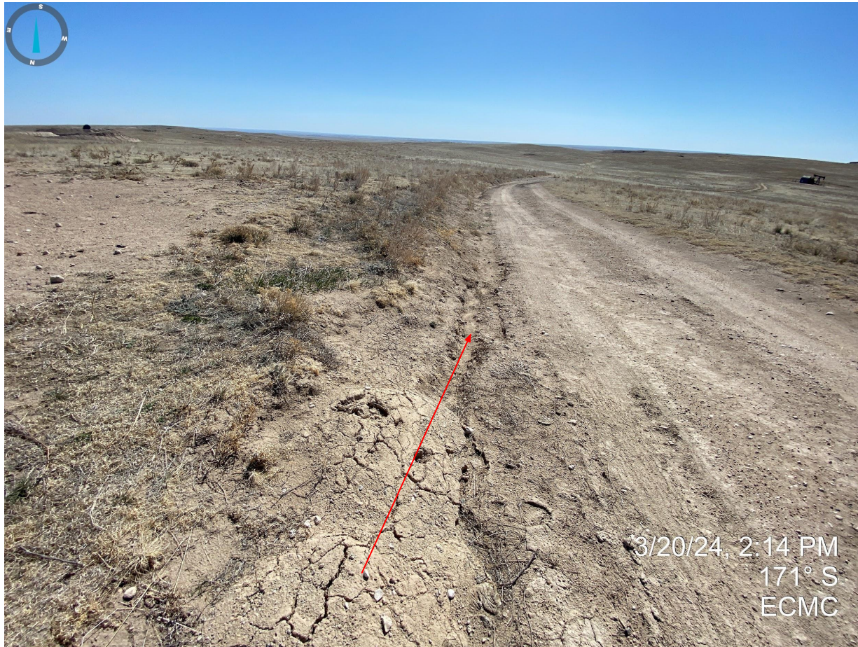
Photo 4. Erosion degradation occurring alongside the access road leading to well API 075-06964.
