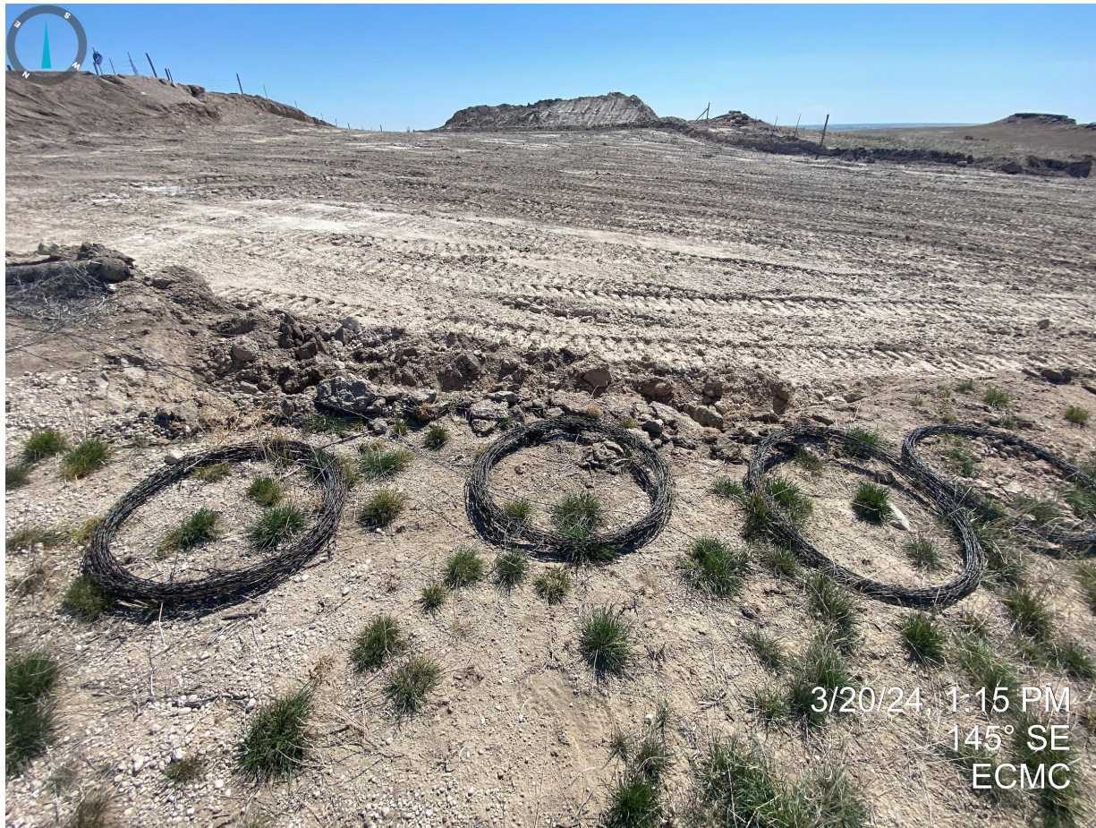
Photo 23. Unused fencing material needs to be removed from the location or returned to service as it poses a potential hazard to personnel, livestock and wildlife resources.
