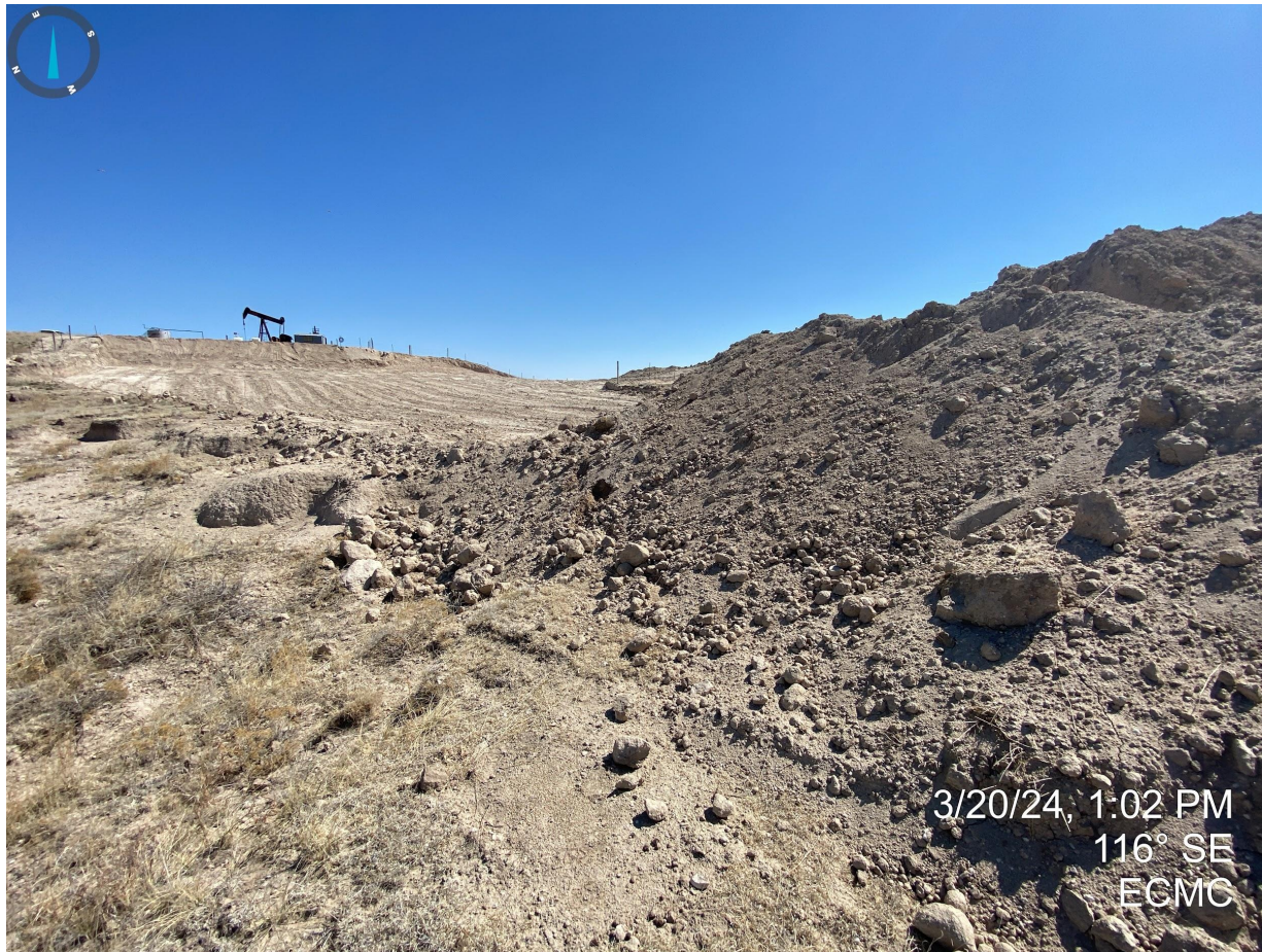
Photo 18. Continued from Photo 17. Photo illustrates unconsolidated materials with no apparent stormwater control measures.
