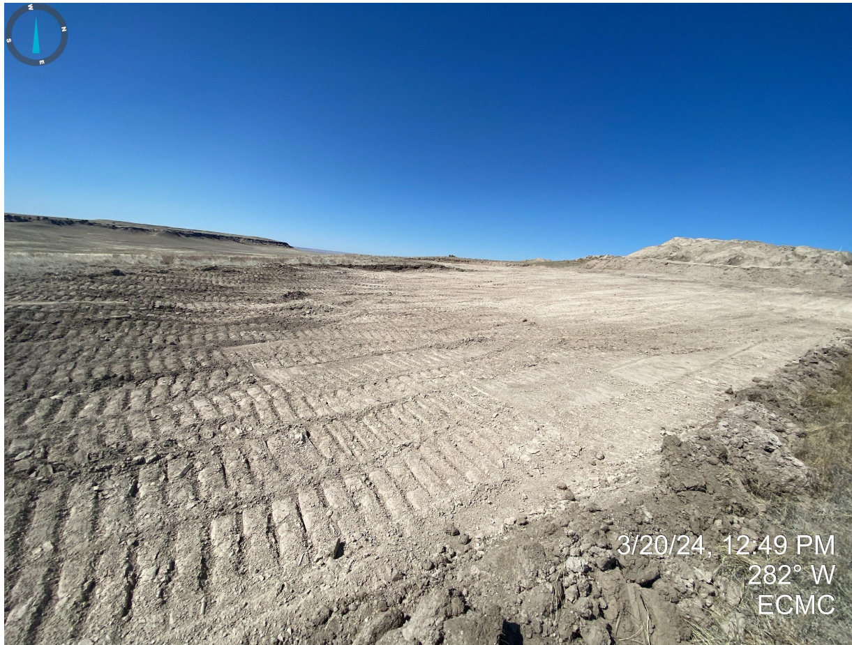
Photo 10. An area approximately 0.50 acres in size has been excavated south of the pit and stockpile. No evidence of stormwater controls measures were observed around the perimeter of the excavated salt kill impacted area.
