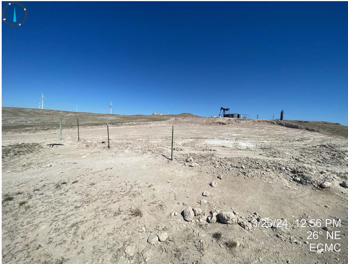
Photo 13. Overview of excavated pit and salt kill area. Soils do not appear to be properly stabilized from wind and water erosion degradation.
