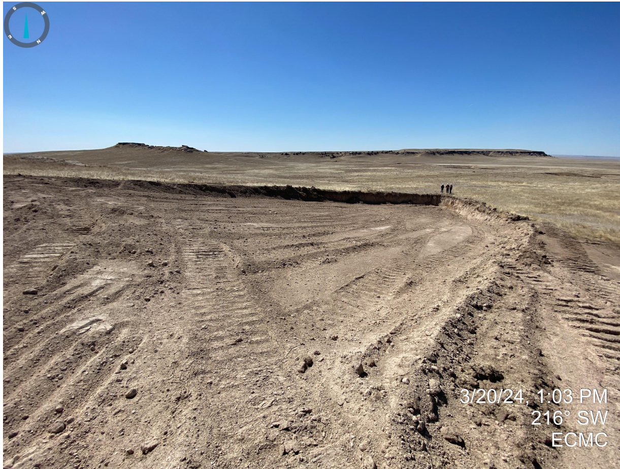
Photo 20. At the time of this inspection, Staff observed a new excavation extending to the western portions of the salt kill impacted area. No apparent stormwater control measures were observed around the perimeter of the excavation and soils have been left unconsolidated.
