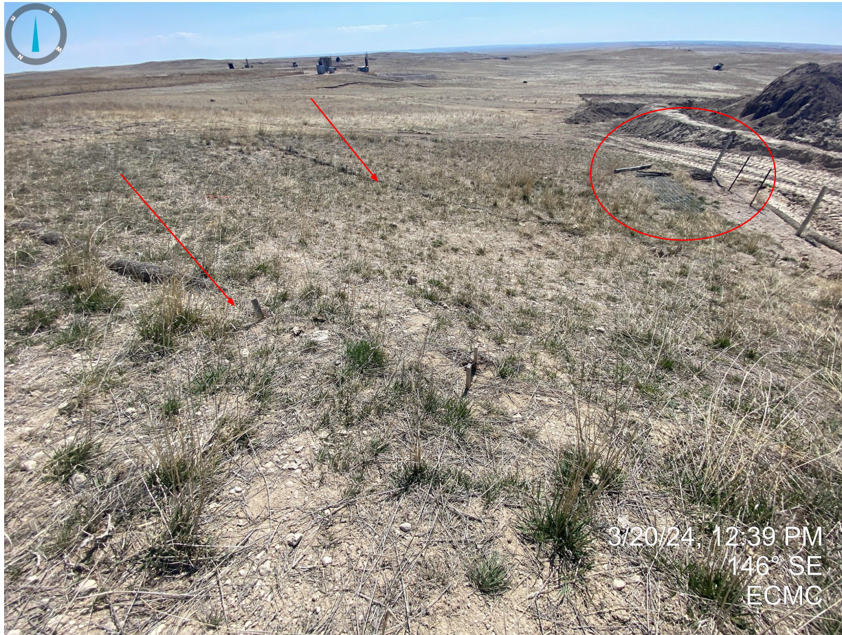
Photo 5. Degraded straw wattles are considered debris as they're beginning to fill with sediment and are no longer adequate or in proper working condition. Also pictured in background (red circle), fencing materials are considered unused equipment and need to be removed or returned to service.
