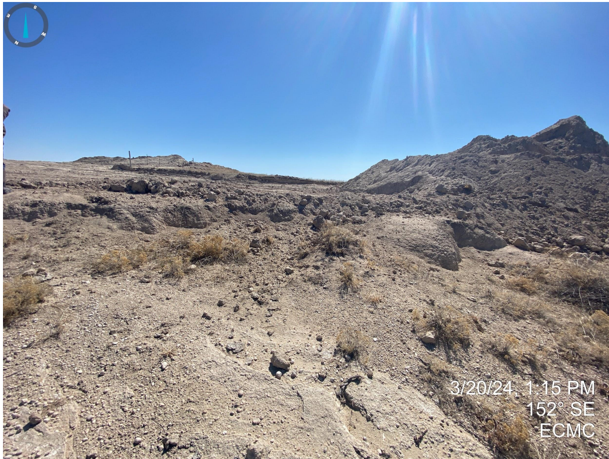
Photo 19. Continued from Photo 17 & 18; taken from nearby drainage. No perimeter stormwater control measures observed around the excavated areas or stockpiled material.
