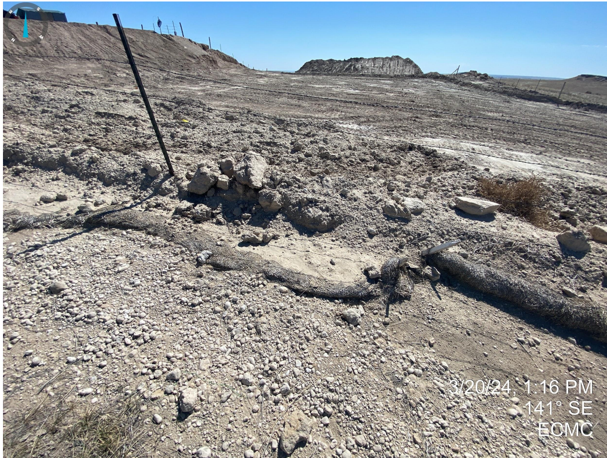
Photo 25. Continued from Photo 24; close up of degraded stormwater BMPs.
