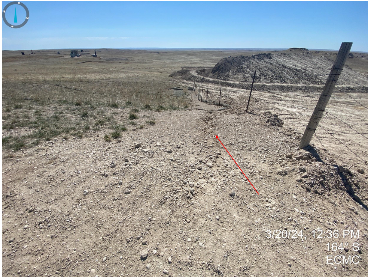
Photo 4. Erosion degradation on the east side of the pit. No stormwater control measures/BMPs observed.
