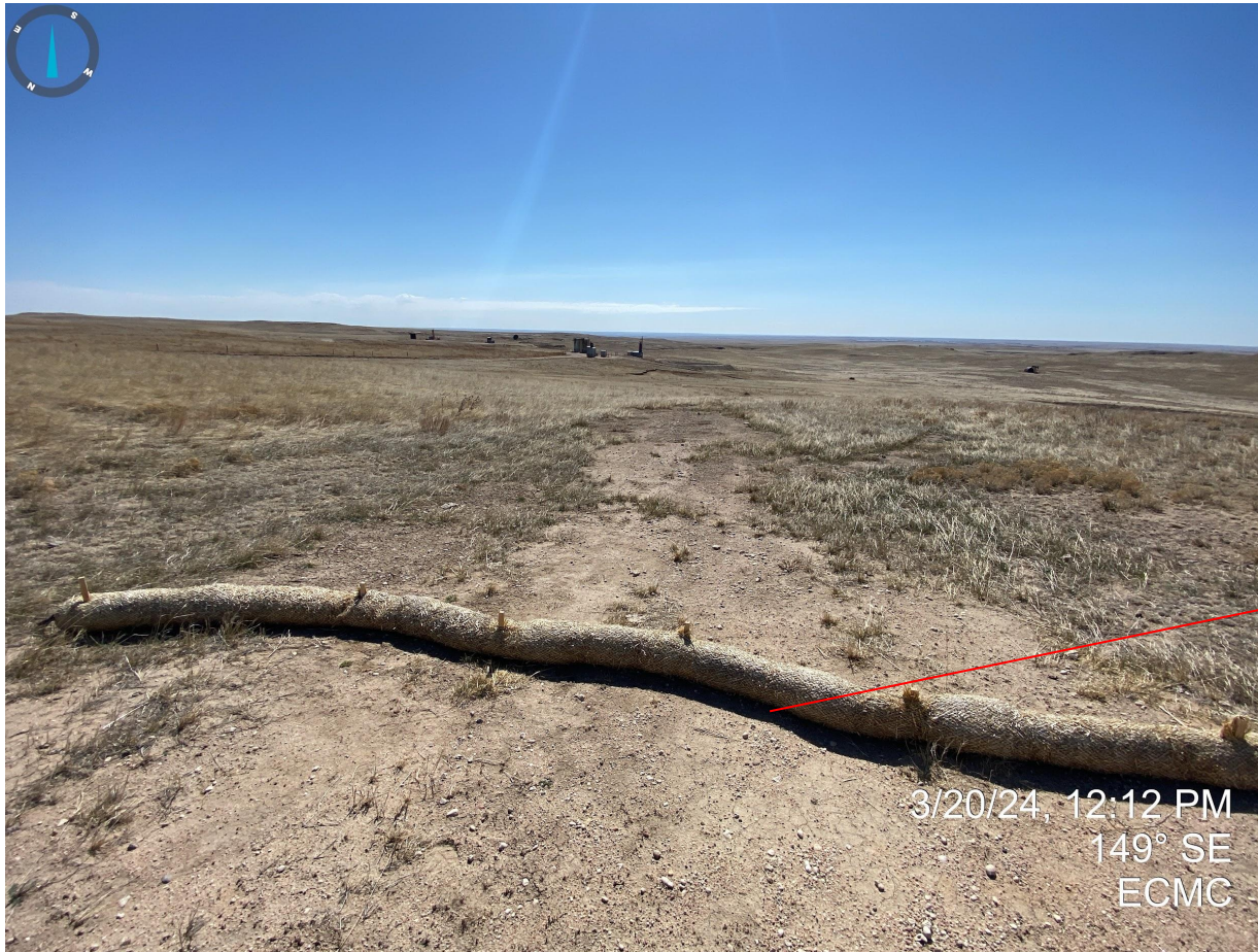
Photo 1. Taken south of the vertical heater treater. Straw wattles have been staked in place but do not appear to be installed per good engineering practices (e.g. trenched and backfilled). Soils remain bare/exposed and are susceptible to wind and water erosion degradation.
