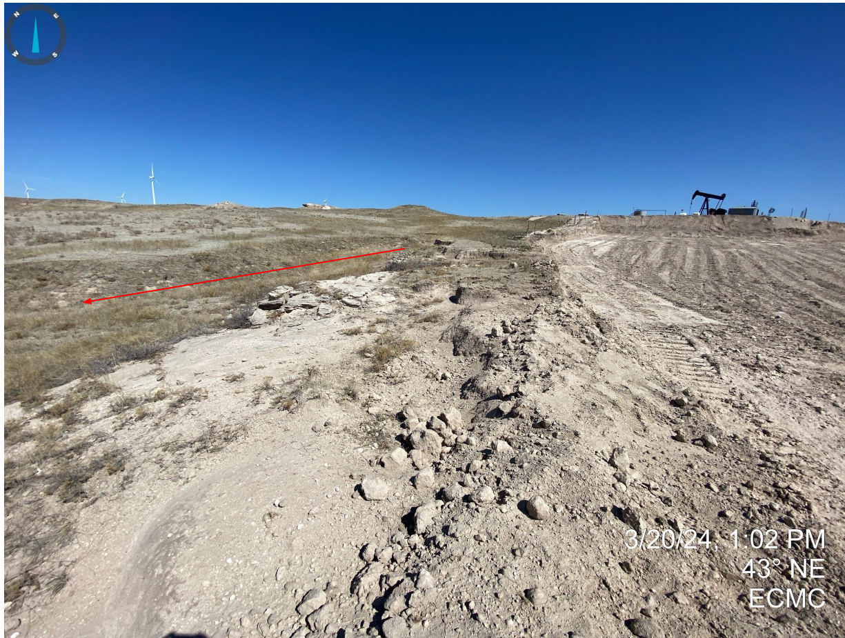
Photo 17. North side of excavation. No stormwater control measures were observed around the perimeter of the excavated area that would prevent off location stormwater discharge from entering nearby drainage (indicated by red arrow).
