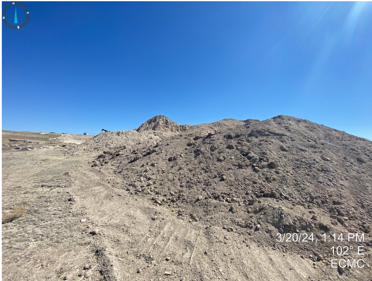
Photo 22. Continued from Photo 21. Western stockpiled material is not properly stabilized with evidence of unconsolidated materials.
