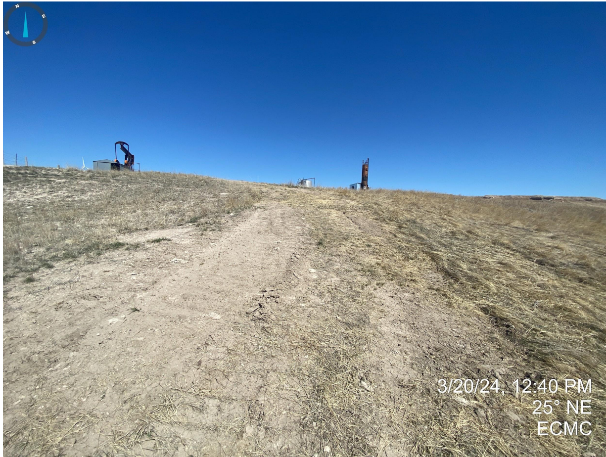
Photo 6. Evidence of vehicle traffic observed east of the pit has left the soil unstabilized; the implementation of stormwater control measures/BMPs and/or reclamation activities are required to prevent erosion degradation.
