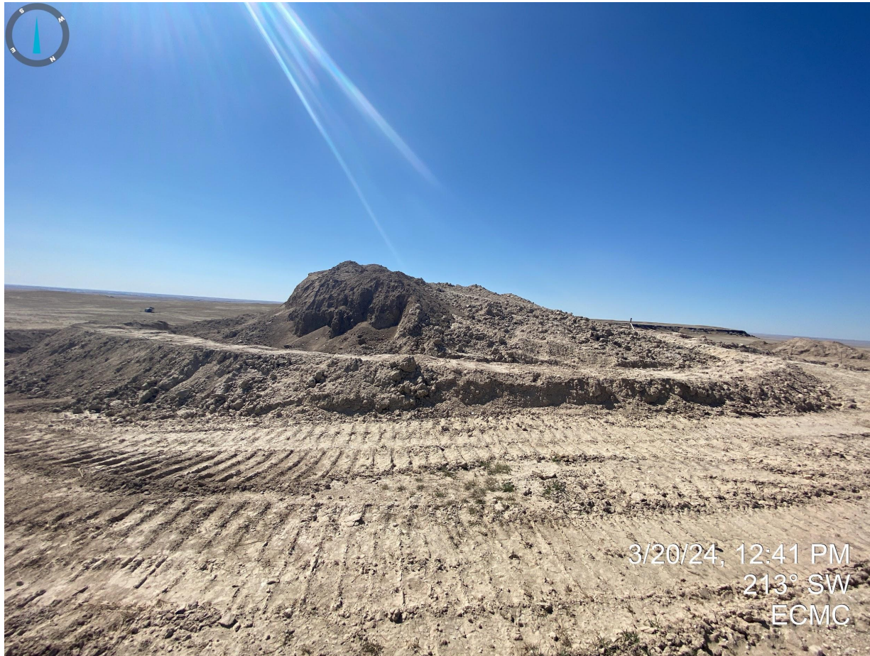
Photo 8. East side of stockpiled pit soils. Photo illustrates that both the stockpile and berms have been left unconsolidated. Unconsolidated materials can become a potential pollution source as it is not properly stabilized.
