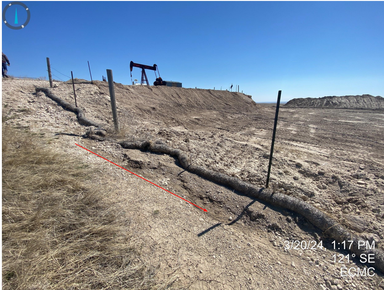
Photo 26. Continued from Photo 24; erosion degradation has not been repaired or stabilized.
