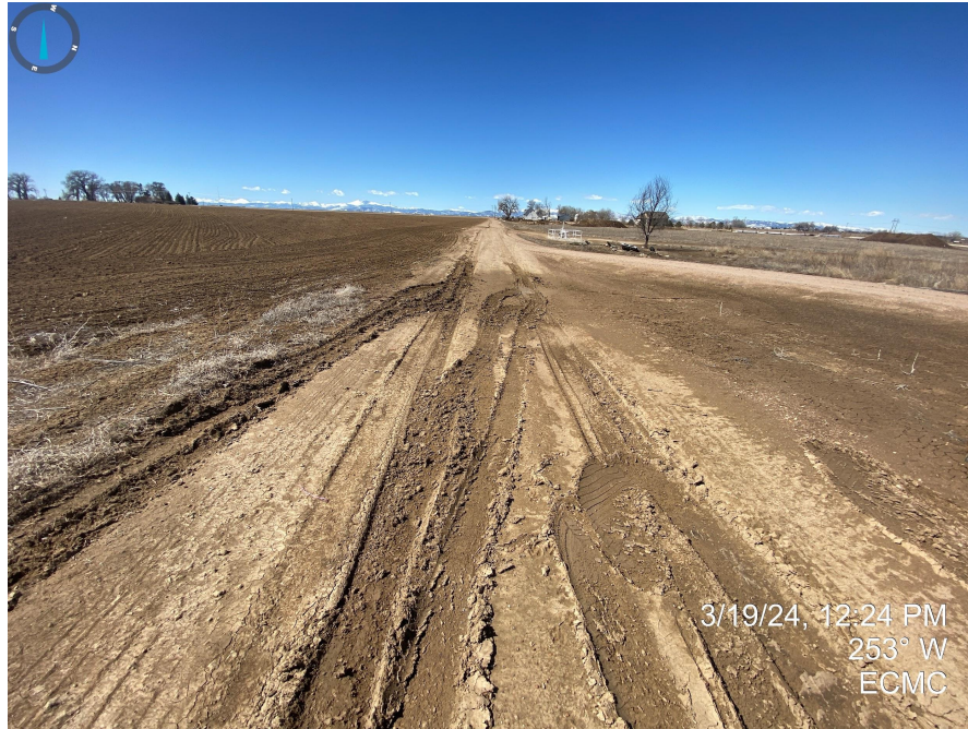
Photos 1 & 2. Taken near the location entrance and access road intersection. Access road requires maintenance as it is beginning to rut which can contribute to vehicle track out.
