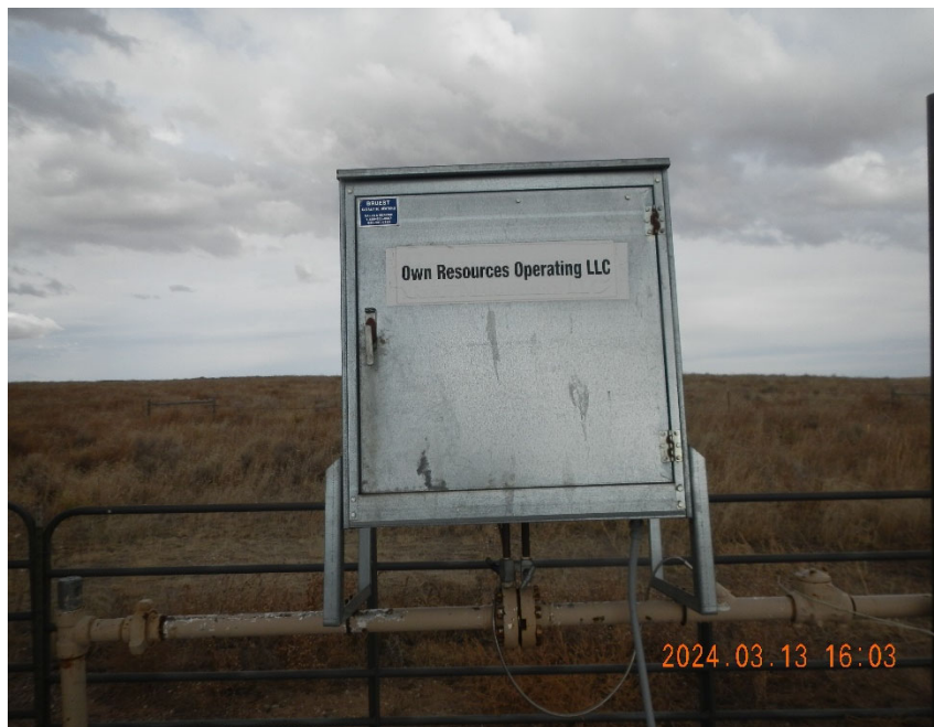
3. Flowline mounted meter box.
