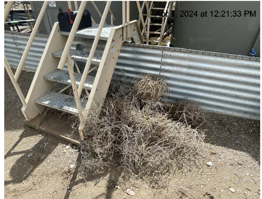
Photo # 2052 Dead weeds/debris
