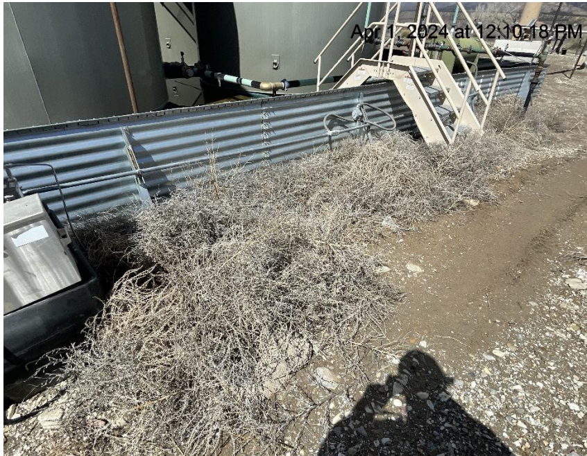
Photo # 2051 Dead weeds/debris
