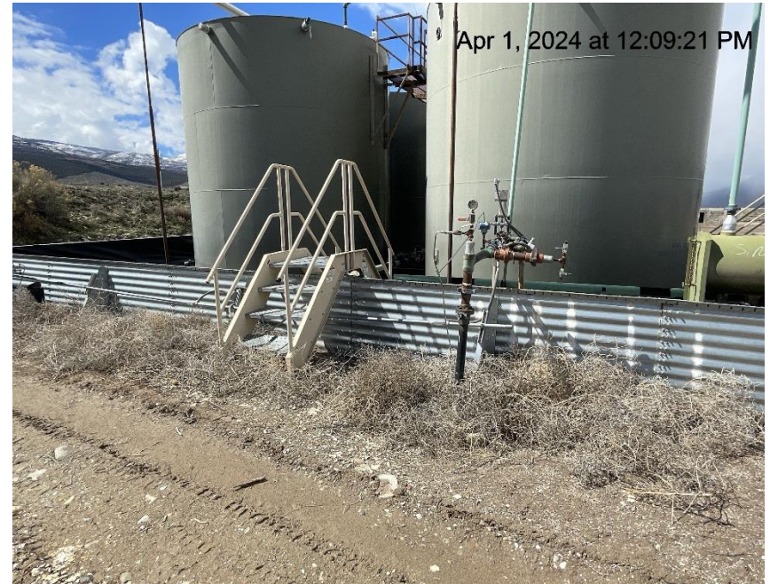
Photo # 2050 Dead weeds/debris
