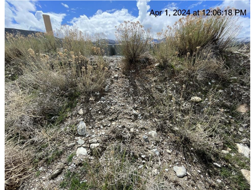
Photo # 2057 Berm/BMP needs maintenance, berm breached/eroded & sediment is being transported off location into a vegetated area. (Berm on north side of location)
