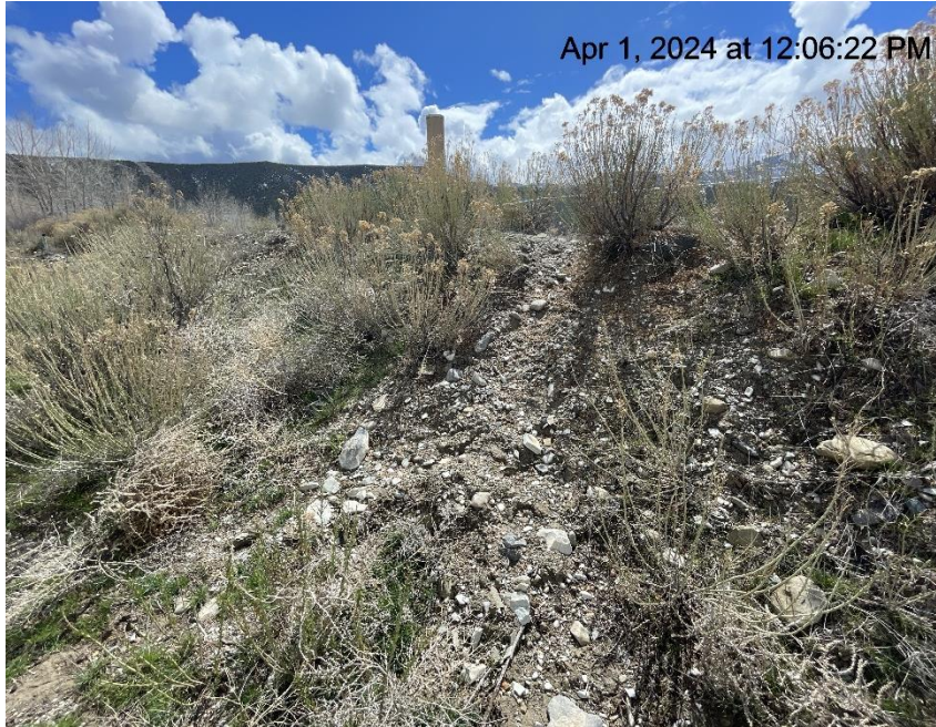
Photo # 2056 Berm/BMP needs maintenance, berm breached/eroded & sediment is being transported off location into a vegetated area. (Berm on north side of location)
