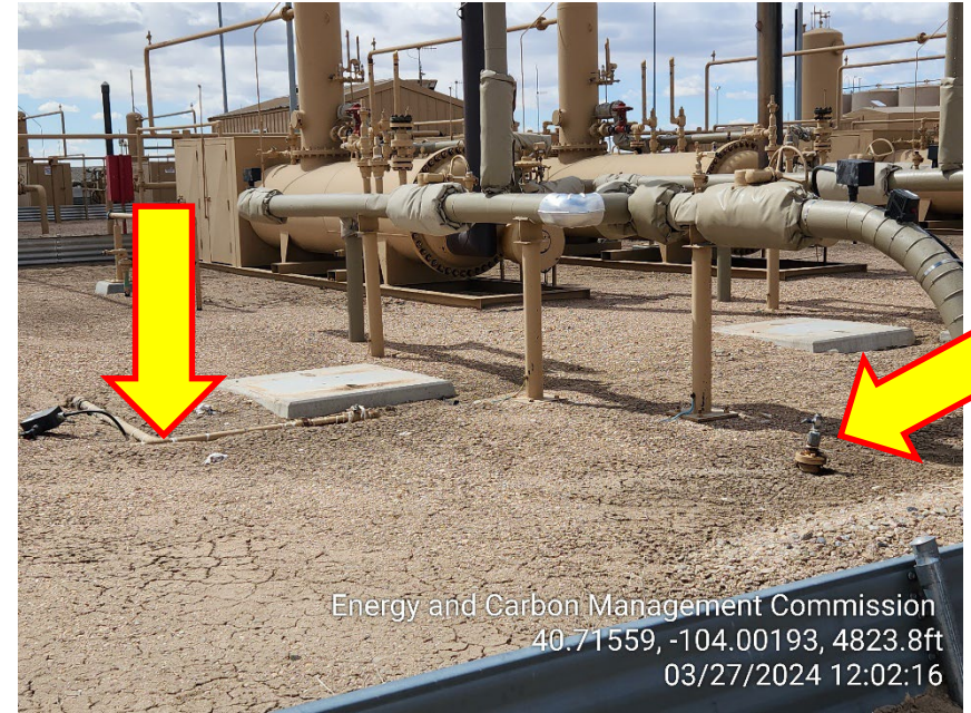
Photo 14 – Unmarked Risers at Separators
