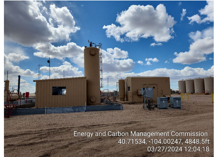
Photo 16 – Heater Treater and Instrumental Air Unit
