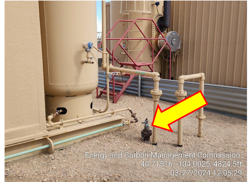
Photo 18 – Unmarked Riser at Air Unit
