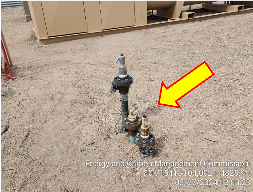
Photo 15 – Unmarked Risers at Separators
