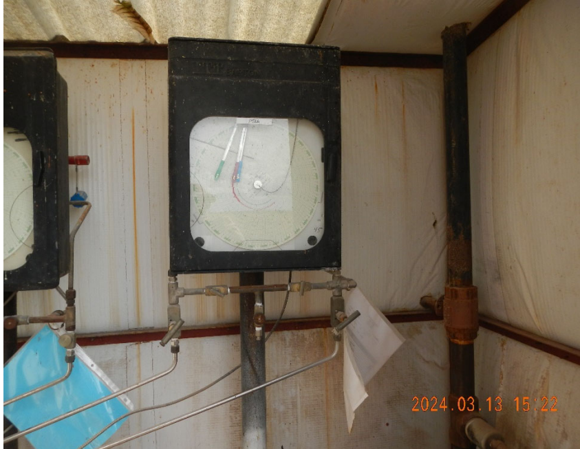
5. Gas meter inside shared meter shed.
