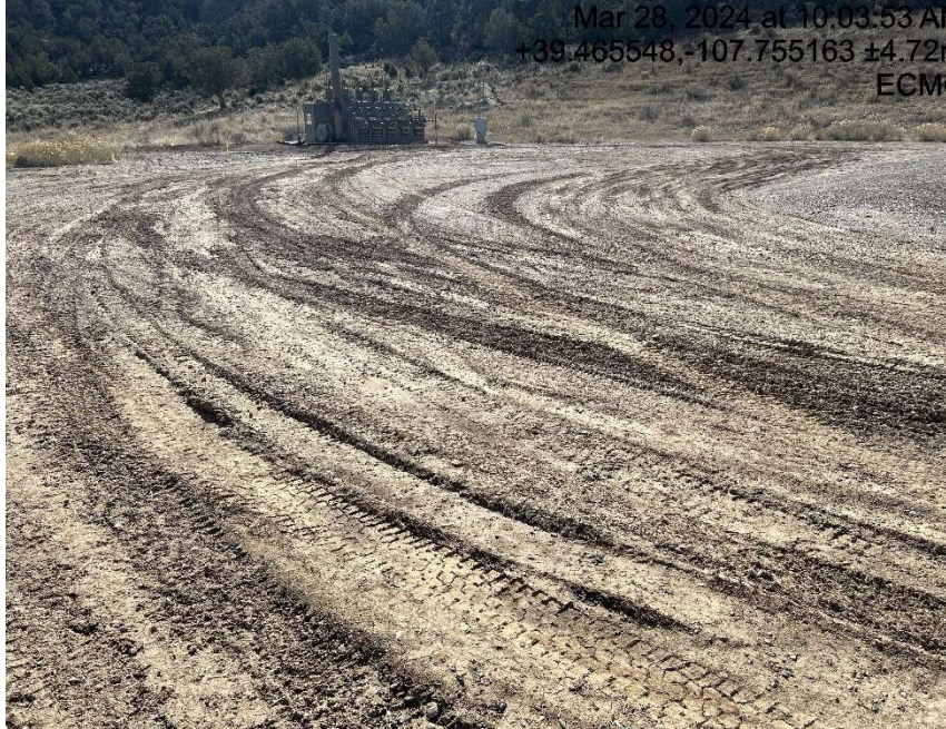
Lack of stabilization/compaction
