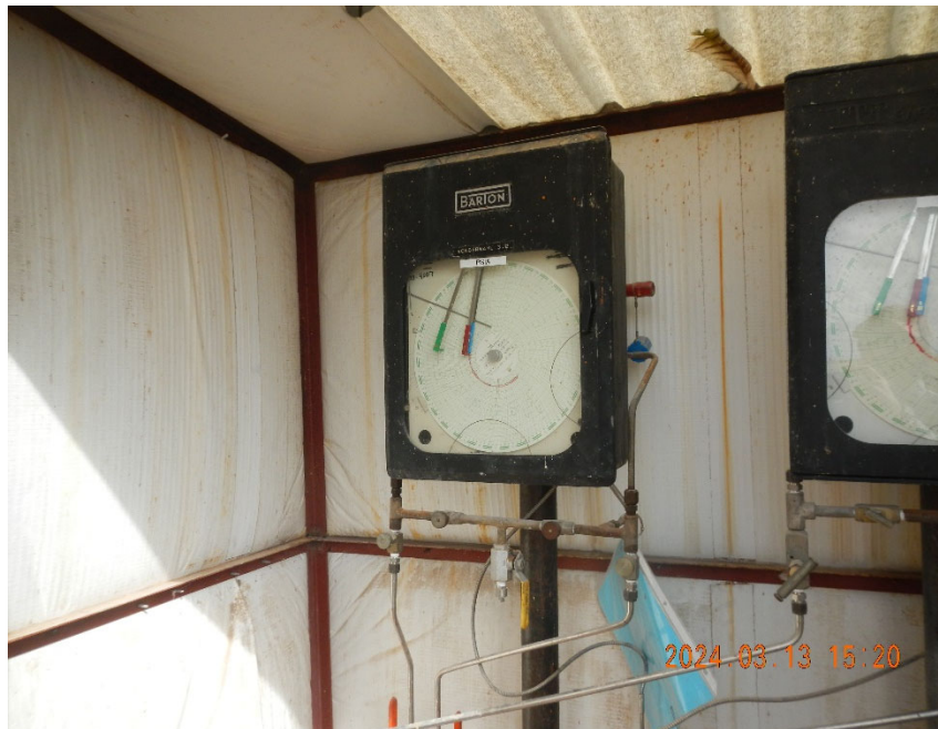
5. Gas meter inside shared meter shed.
