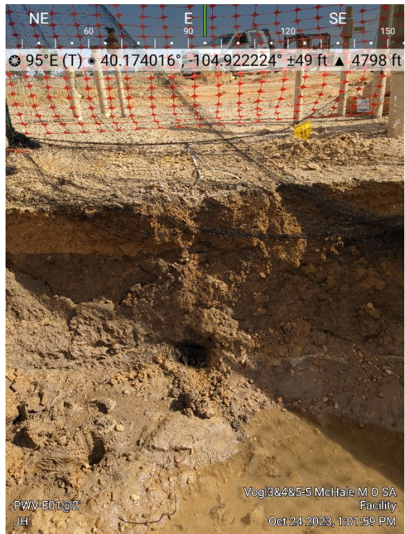
PWV Excavation (Groundwater present in excavation)
