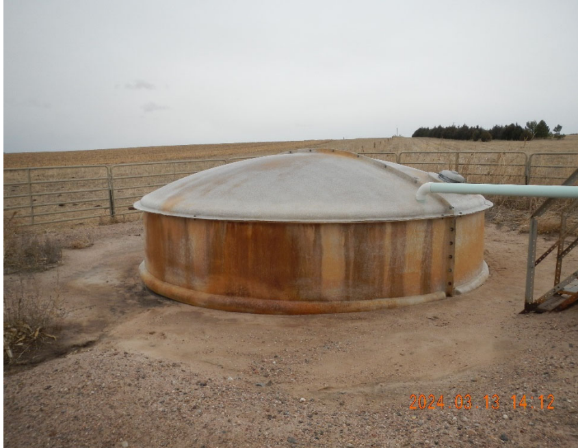
7. View of produced water tank.
