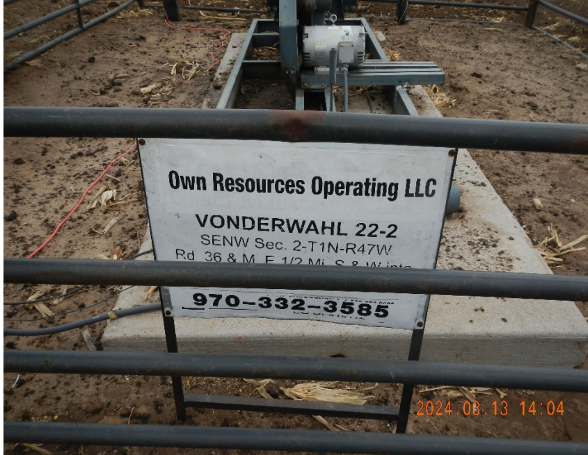
1. Well sign at well location.
