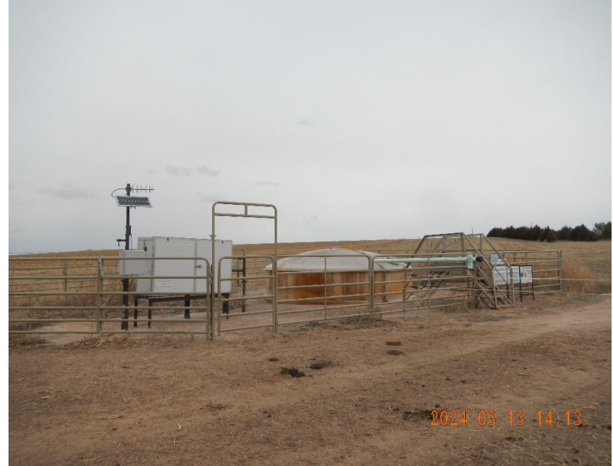
8. Remote metering location overview.
