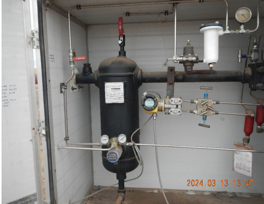
5. View of separator and digital gas meter inside meter box.
