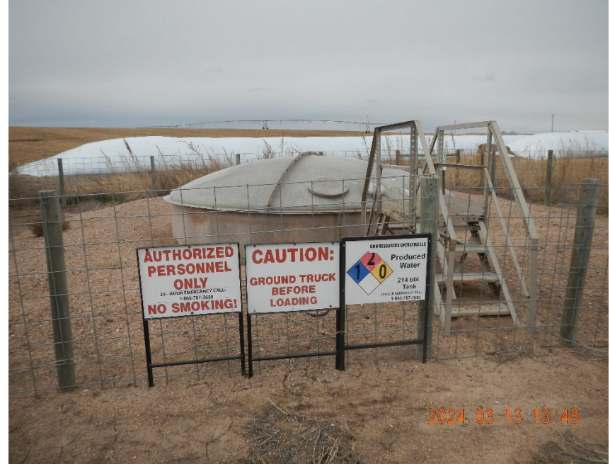
6. Produced water tank and signage.
