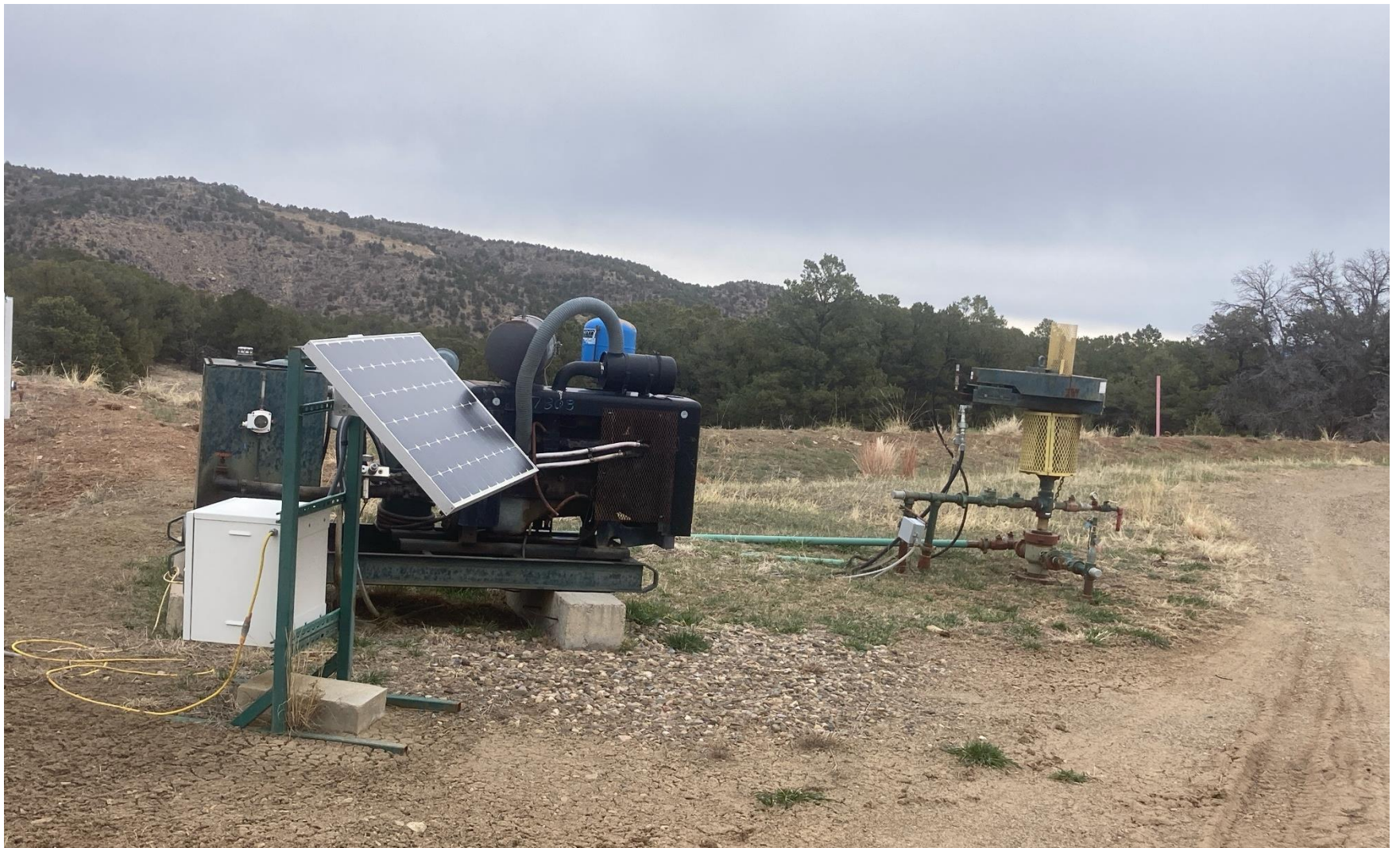
PHOTO 3: TR WELLHEAD AND EQUIPMENT
