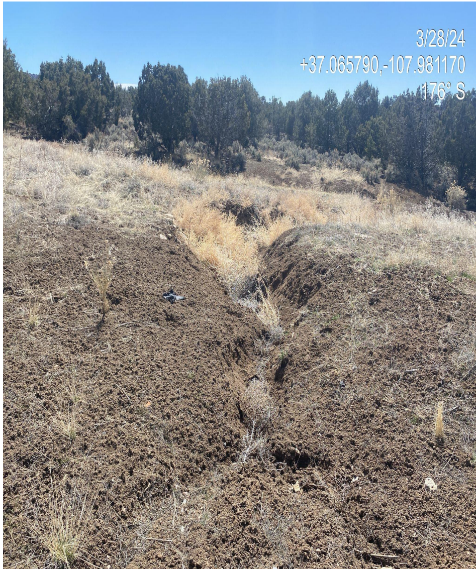
Photo 4. View of gully erosion observed forming in the southwest corner of the disturbance. Current stormwater BMPs are not adequate.
