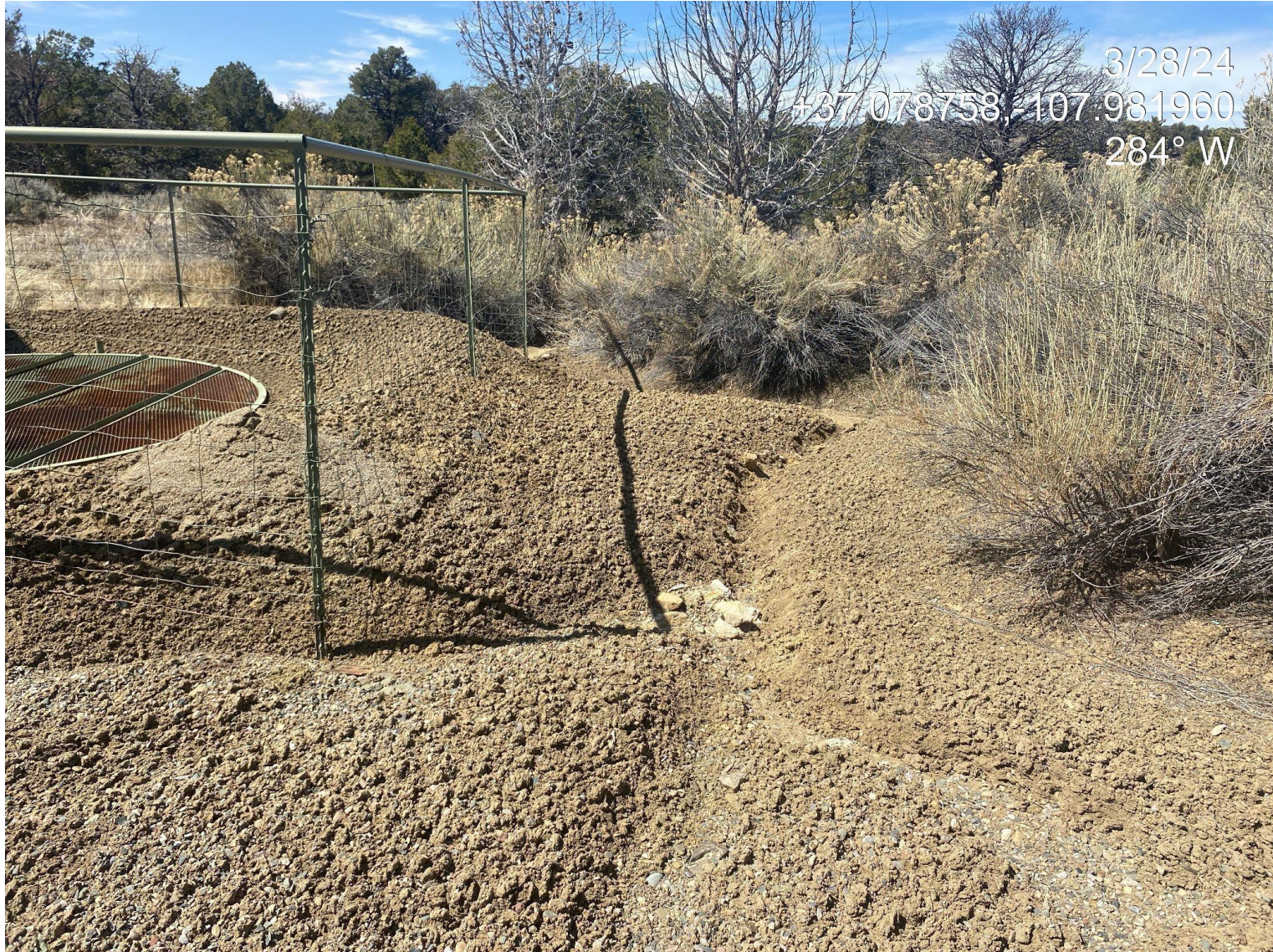
Photo 4. Rill erosion observed forming along the fence line of the produced water tank.
