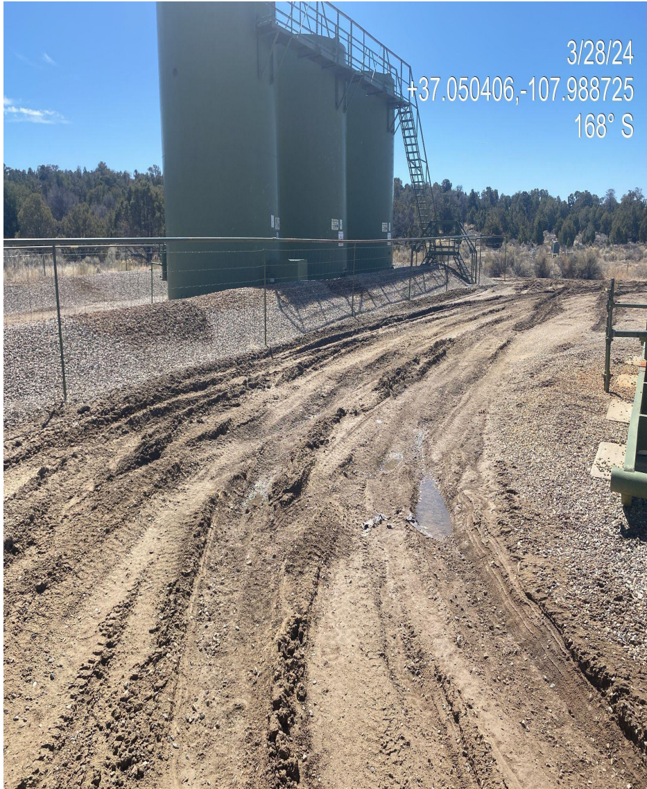
Photo 3. Rutting observed in the southern portion of the disturbance. Additional stabilization is needed to minimize stormwater and site degradation.
