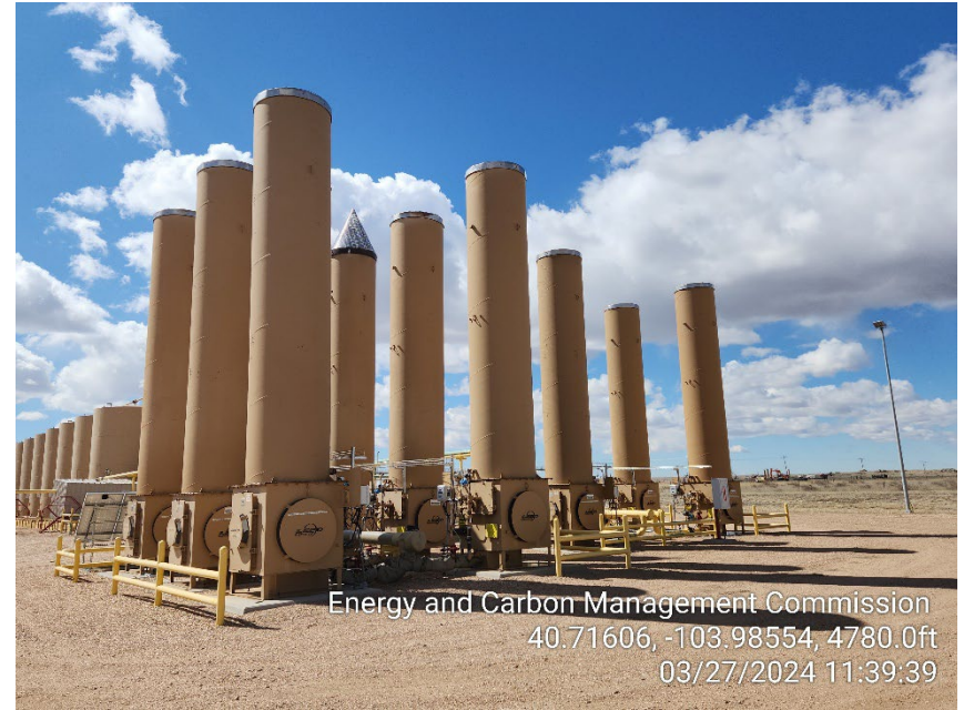
Photo 18 – Crude Oil Tank ECDs
