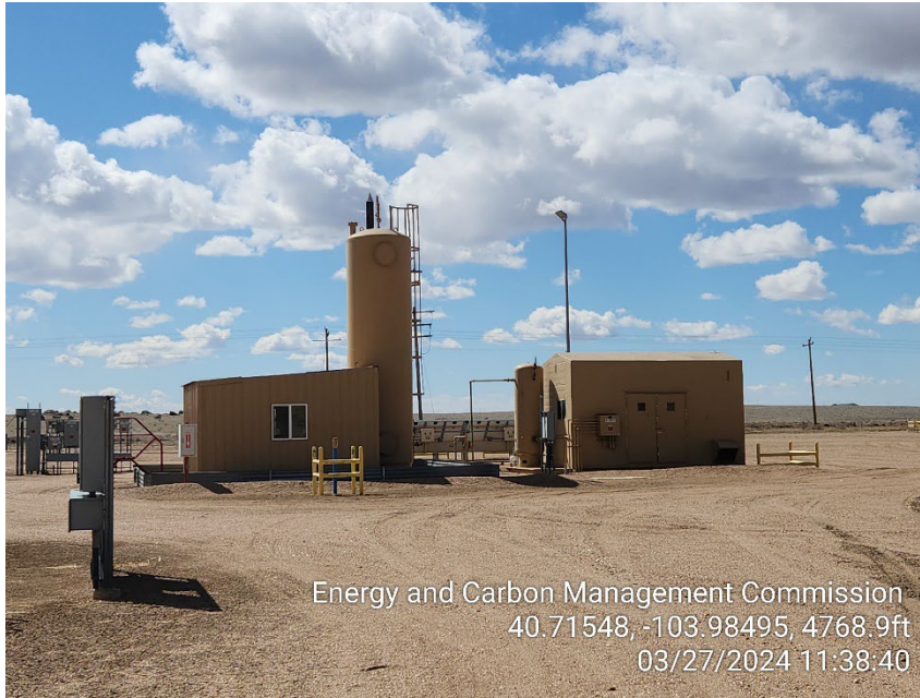
Photo 15 – Heater Treater and Instrumental Air Unit
