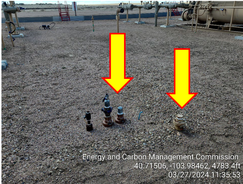
Photo 11 – Risers at South Separators Unmarked
