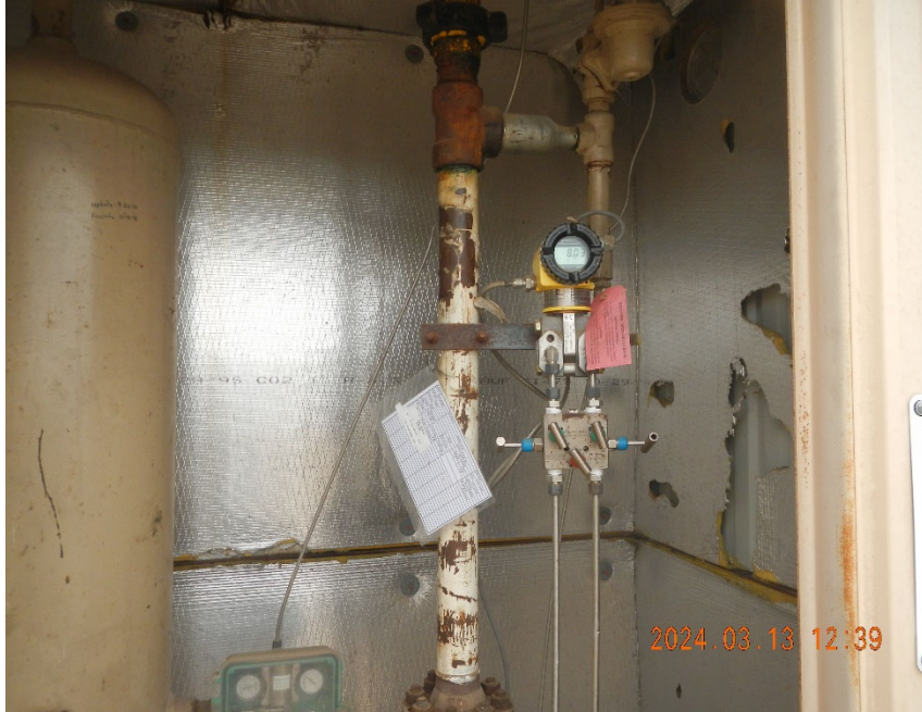
5. Digital gas meter and separator inside meter shed.
