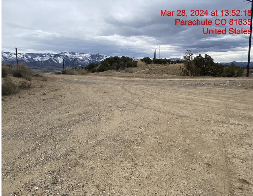
Insufficient Vehicle Tracking BMPs at Location Entrance/Exit – Photo #00238
