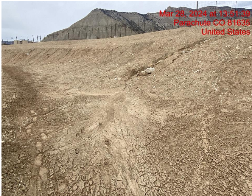
Insufficient Erosion Control – Photo #00236
