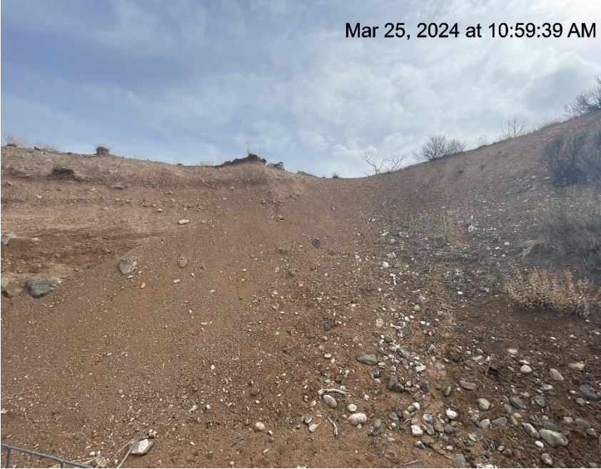
Photo # 1197 Lack of stabilization on cut slope
