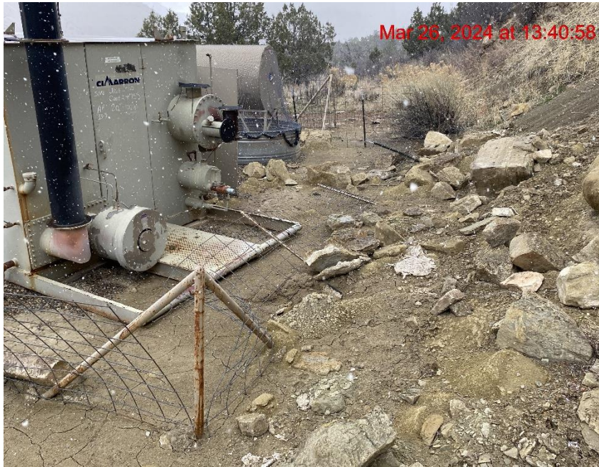
Insufficient Erosion Control/Degradation – Photo #00183
