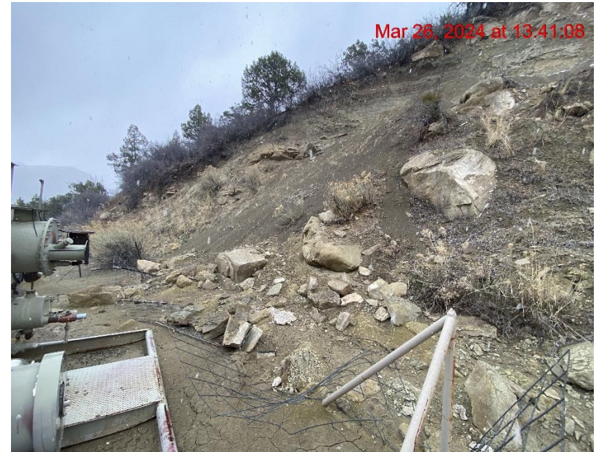
Insufficient Erosion Control/Degradation – Photo #00184
