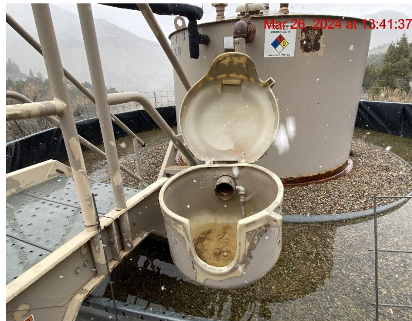
Open-Ended Load Line – Photo #00186
