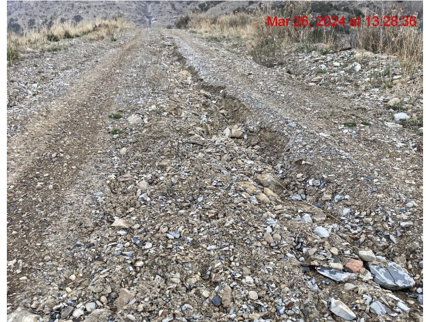
Insufficient Erosion Control – Photo #00169
