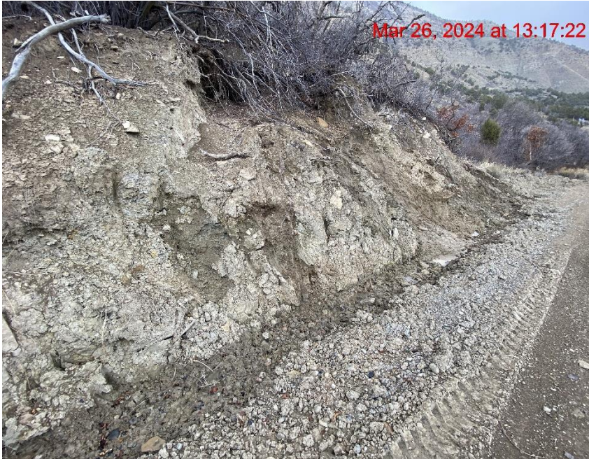
Insufficient Erosion Control on Lease Road Cut Slopes – Photo #00155
