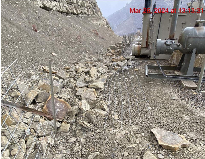
Insufficient Erosion Control/Degradation – Photo #00150
