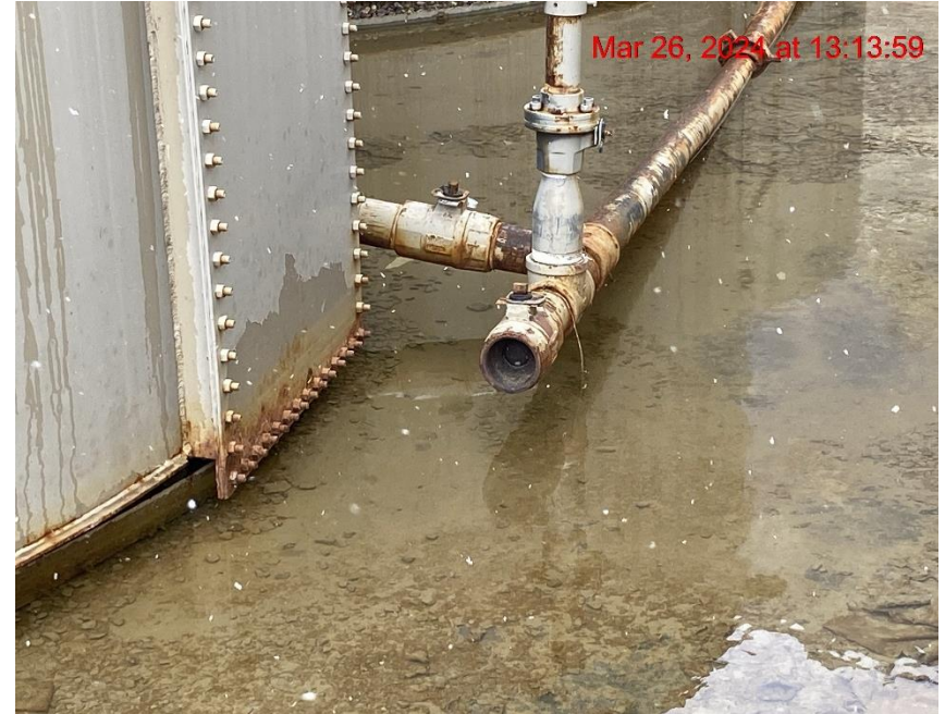
Open-Ended Line in Tank Battery – Photo #00153
