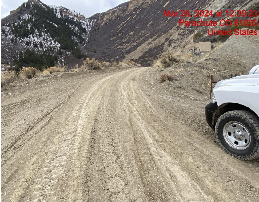
Insufficient Vehicle Tracking BMPs at Location Entrance/Exit – Photo #00118
