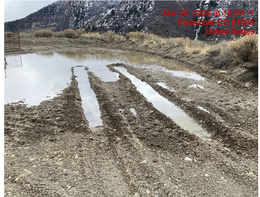
Lack of Stabilization/Degradation – Photo #00117
