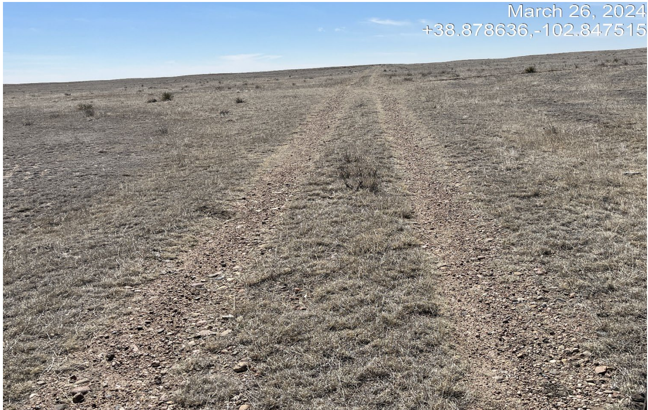
Photo 2. Facing south along the access road. The two track access road remains and will need to be decompacted. Consider decompacted only to two track portion to save vegetated areas.
