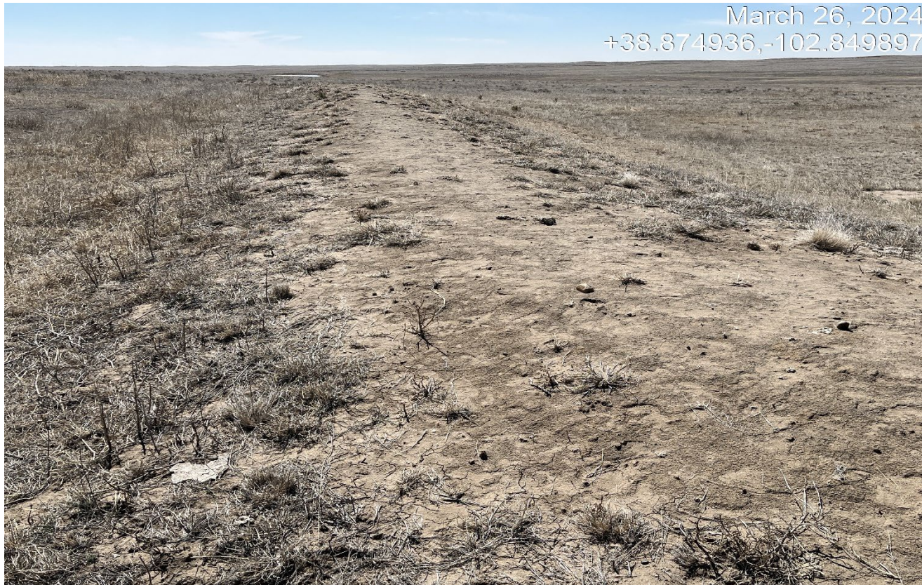
Photo 8. Facing south at the top of the cut slope. There is a berm along the top of the which needs to be recontoured along the cut slope.
