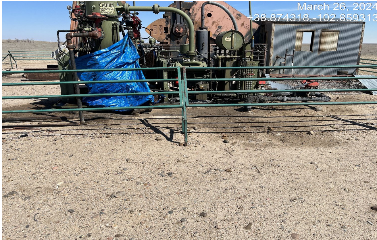
Photo 3. There is stained soils around the engine that needs to be cleaned up.
