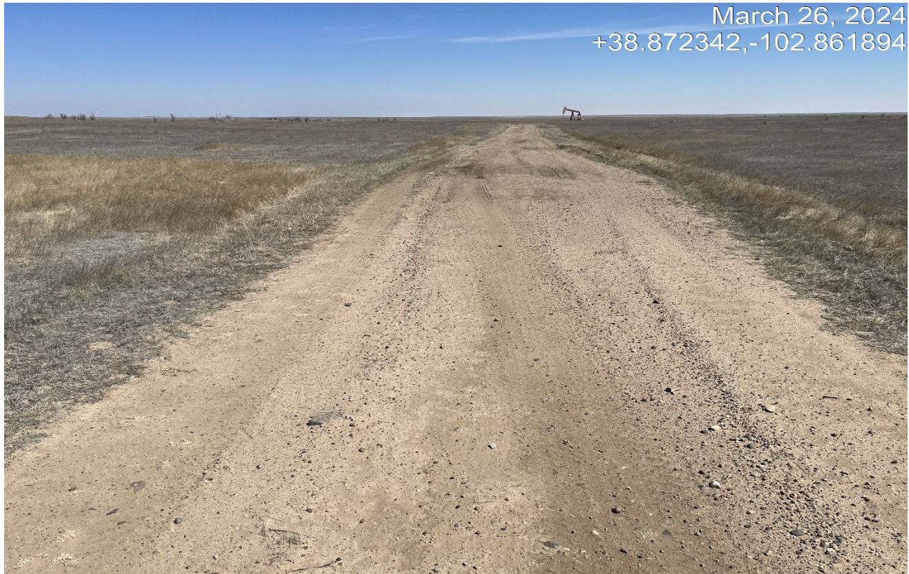
Photo 1. There is road damage which vehicle are avoid which is widening the road.
