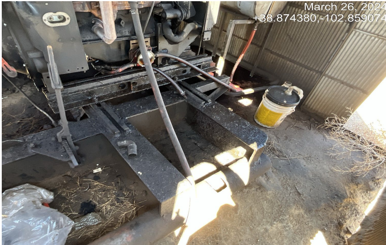
Photo 5. There is oil stained soils from the engine which appears to have leaked for a duration of time.
