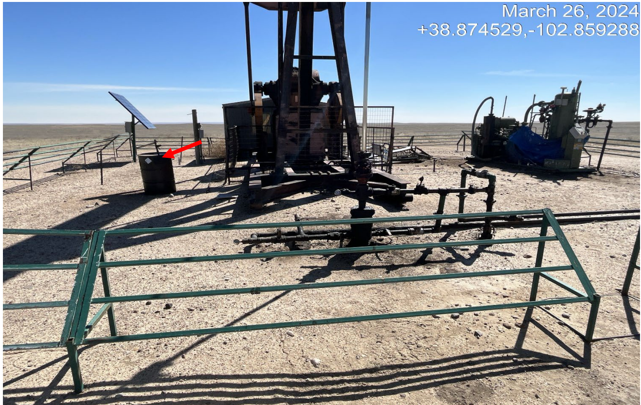
Photo 6. There is a fuel or chemical barrel with no secondary containment.
