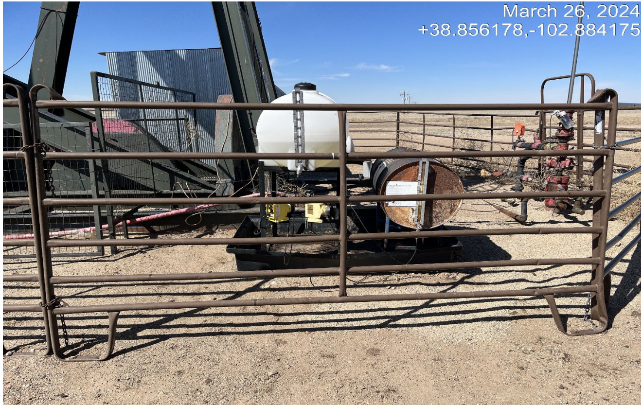
Photo 3. The secondary containment has been cleaned out and weeds removed..
