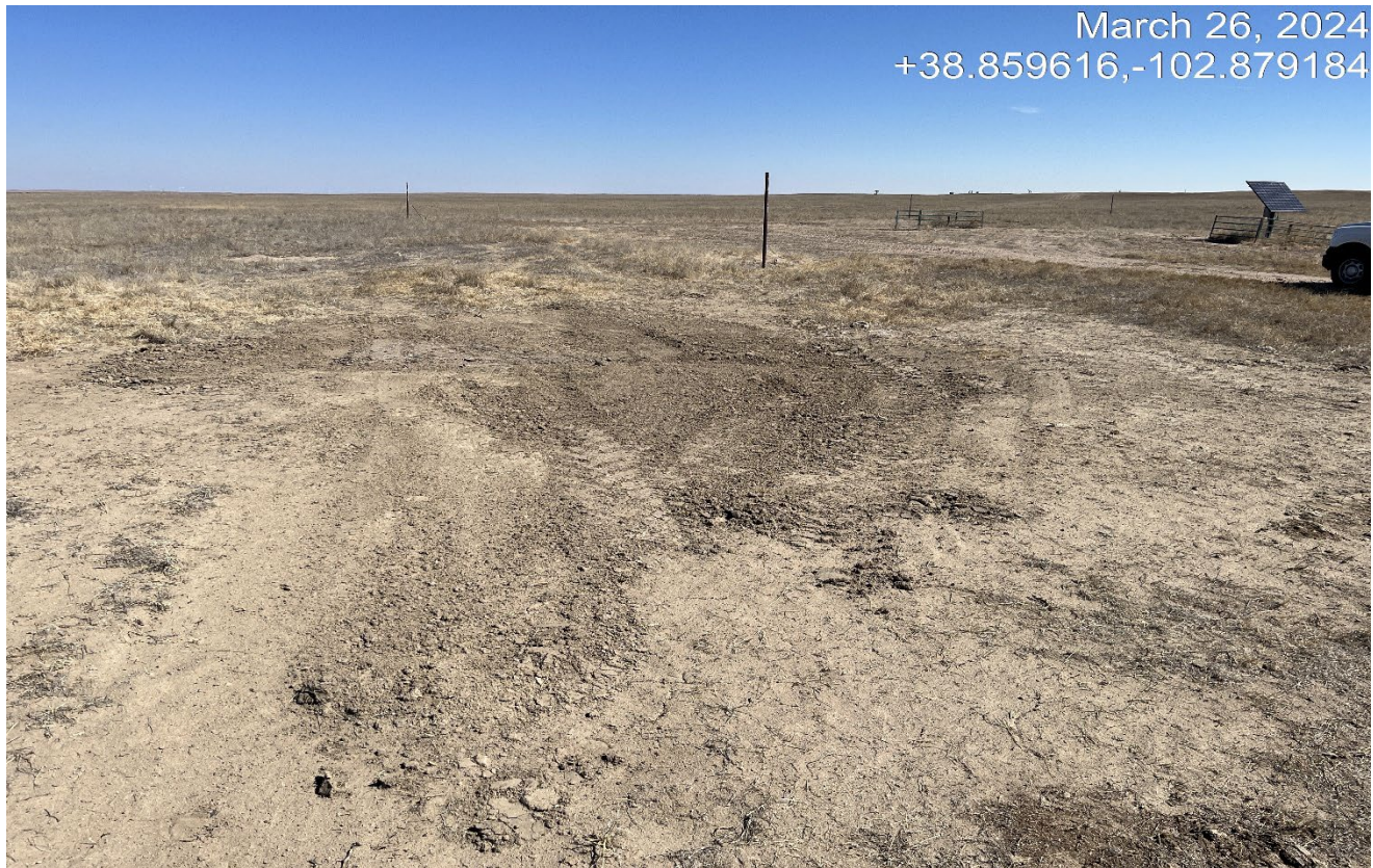
Photo 4. Southwest side of the location facing northeast. There is a pipeline cellar has been removed since previous inspection. The disturbed area will need to be reclaimed.
