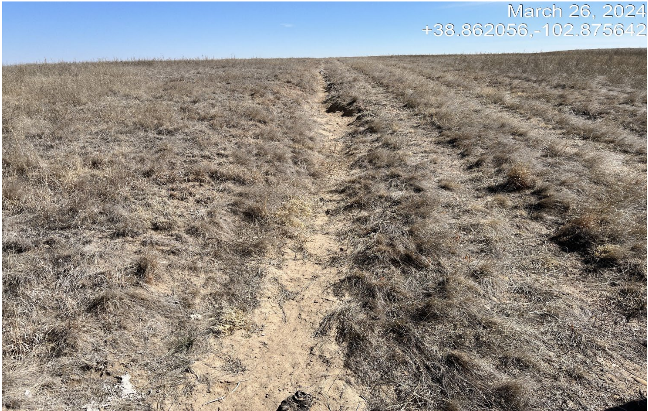
Photo 21. Facing northeast along the two track access road. There is an erosion channel along the road closer to the location that needs to be repaired.
