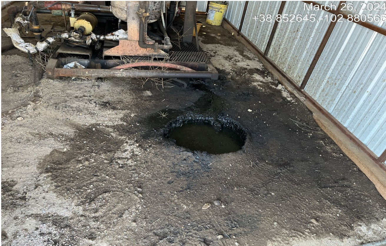
Photo 4. View of inside the shed shows a leak occurring from the pumpjack engine. This needs to be controlled and cleaned up.
