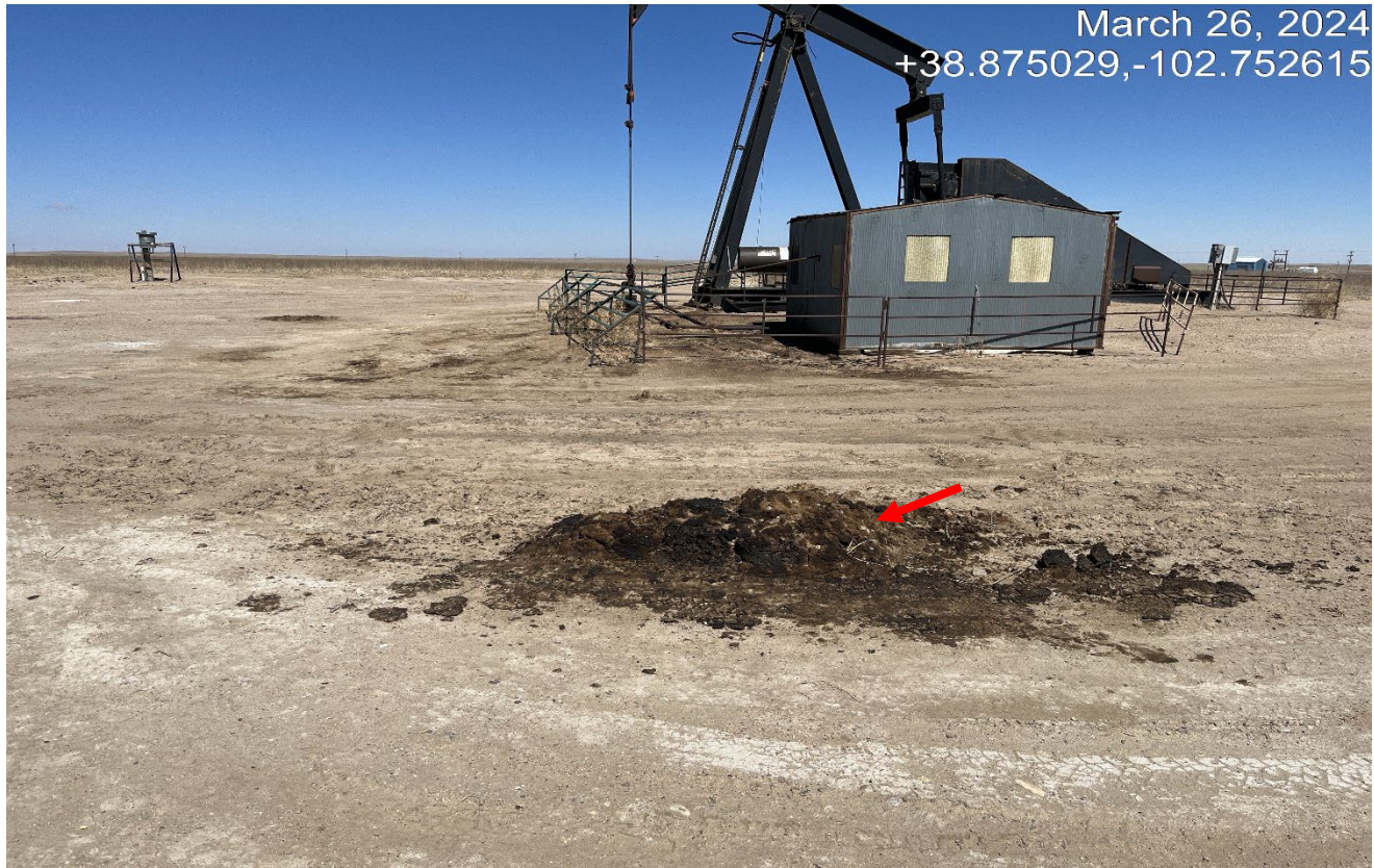
Photo 2. There is a pile of oily E&P waste at the south side of the well. It appears there was a leak at the well and impacted material has not been cleaned and there are even vehicle track thru the oily waste pile.
