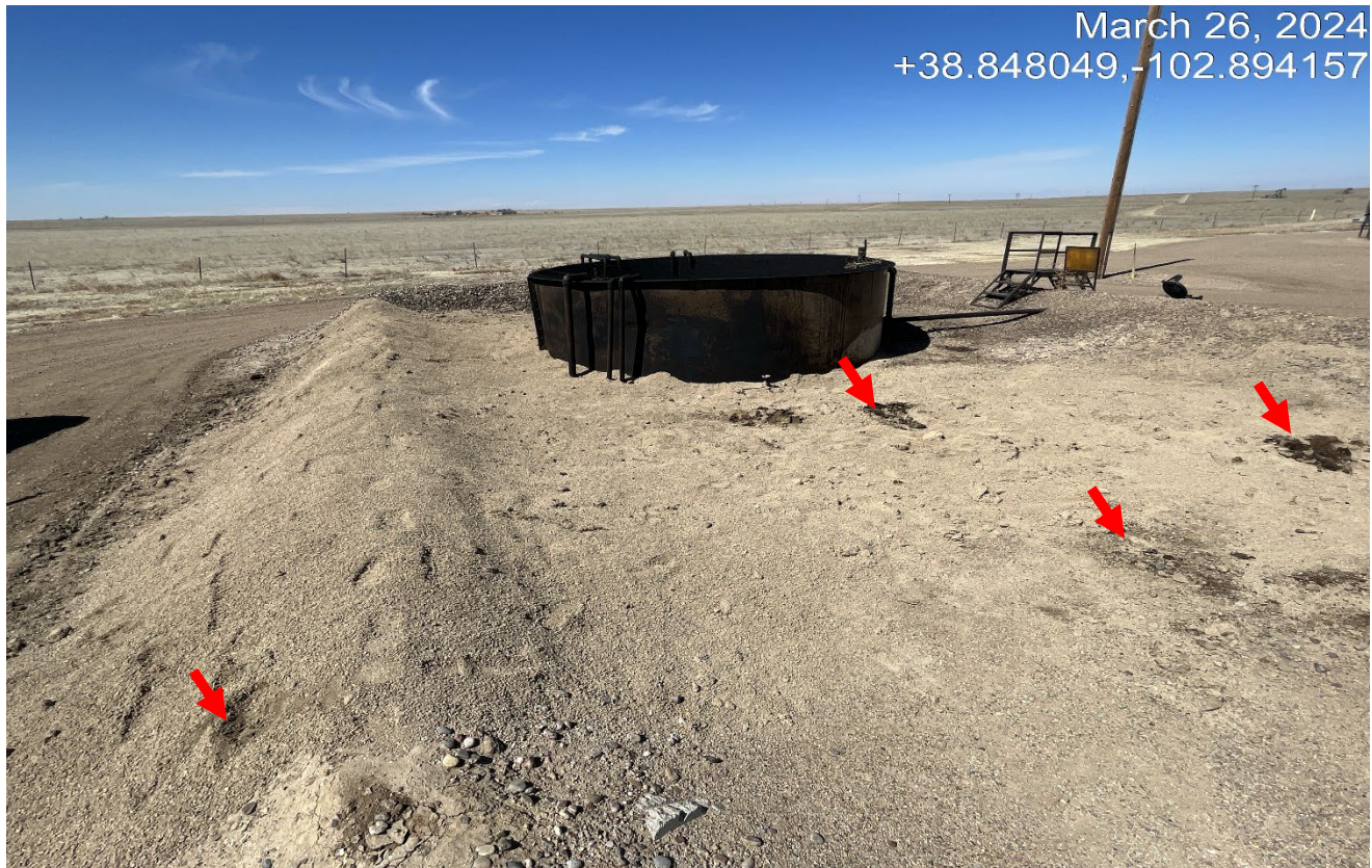
Photo 8. The red arrows point to areas where oily soils have not been cleaned up.
