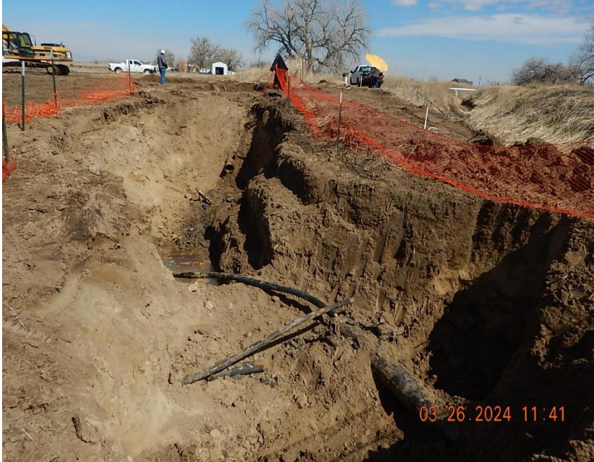
Flowline pipe observed in the south excavation; photo looking north.
