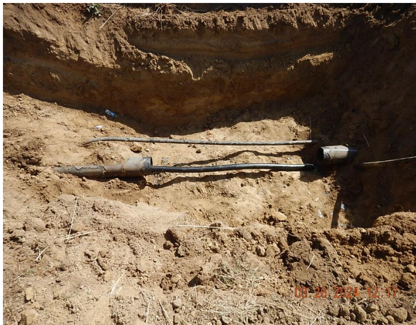
Closer view of flowline pipe observed in north excavation. 3" HDPE poly flowline can be seen entering the cuts end of the 8" carbon steel facility 8 flowline (OOS). In addition, historically AIP 2" CS flowlines were found in excavation.
