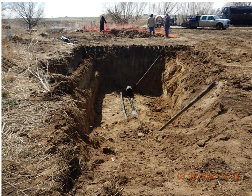
North excavation and flowline pipe exposed. View looking south to excavation where release point identified.
