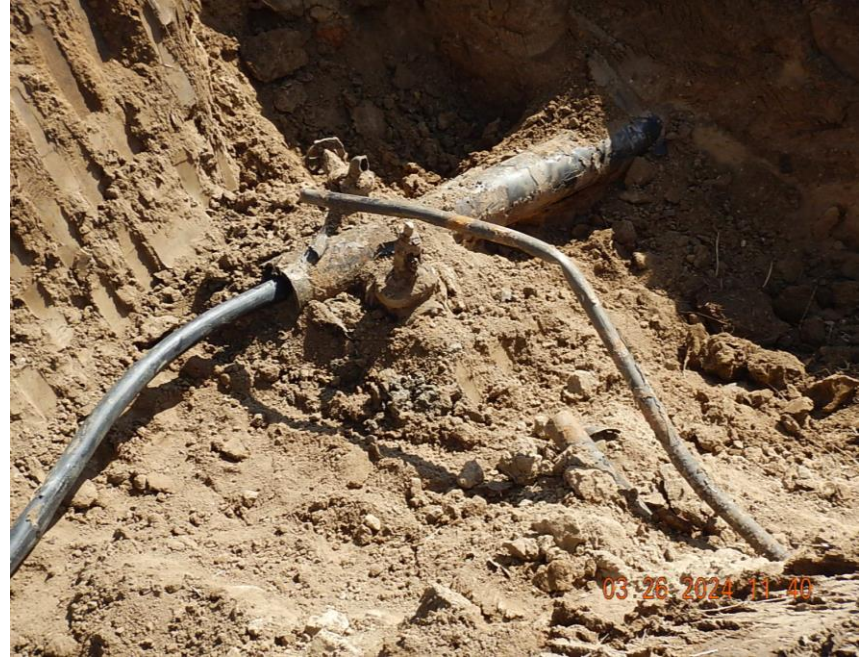
Close up view of flowline pipe exposed in the south excavation; 3" HDPE flowline can be seen entering the cut end of the 8" carbon steel facility 8 flowline (slip line repair). Also, 2" and 4" historically AIP flowlines (and associated tie in valves) observed in the excavation.
