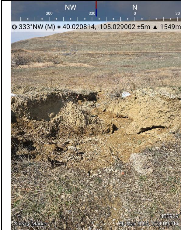
Survey marker at northwest corner of MLVT Pad – 40.020814 / -105.029002
