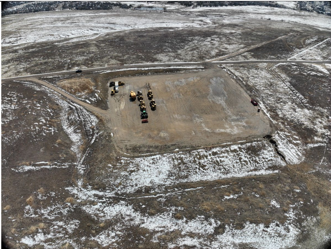
In View – MLVT Pad, Access Road
