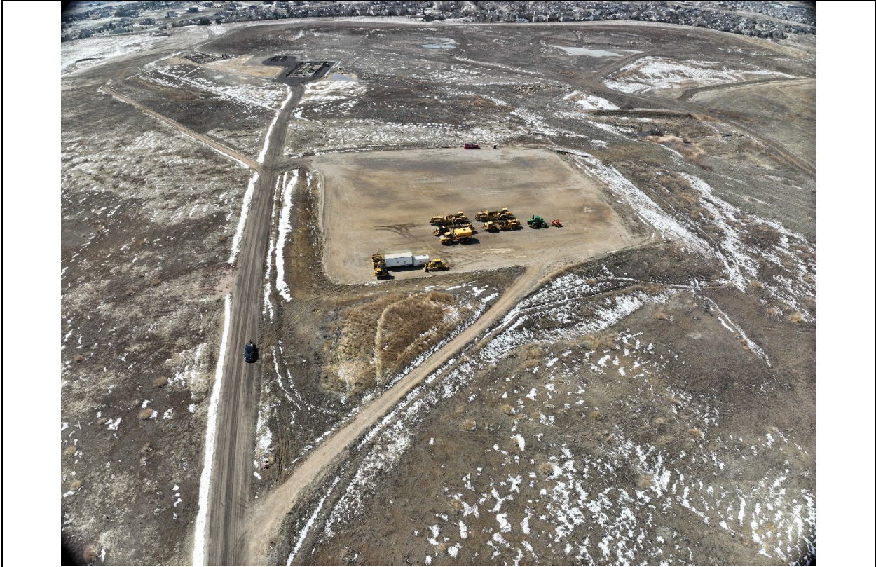
In View – MLVT Pad, Access Road
