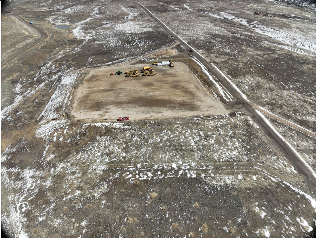
In View – MLVT Pad, Access Road
