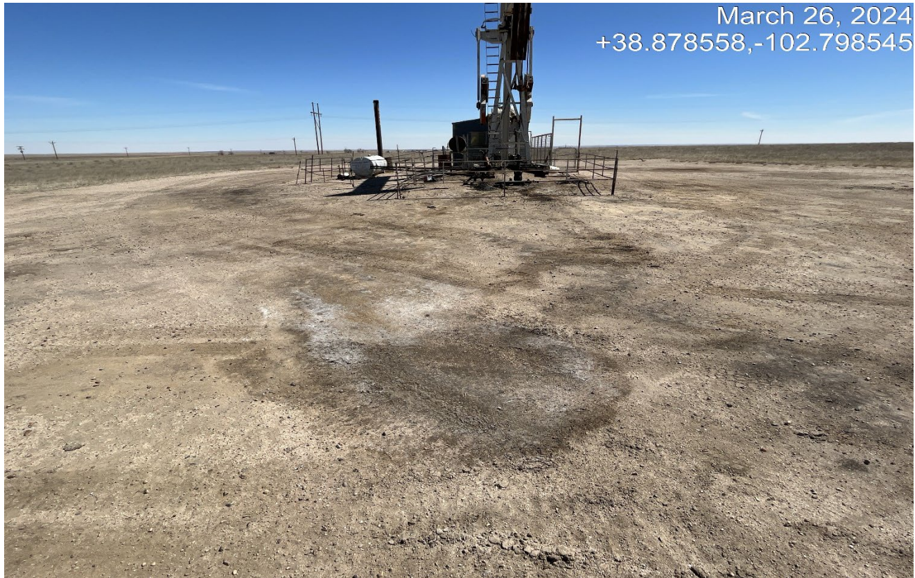
Photo 4. Facing east toward the well. There is signs the a spill occurred at the wellsite that spread out west and south of the well with an undetermined amount spilled which will require a spill report.
