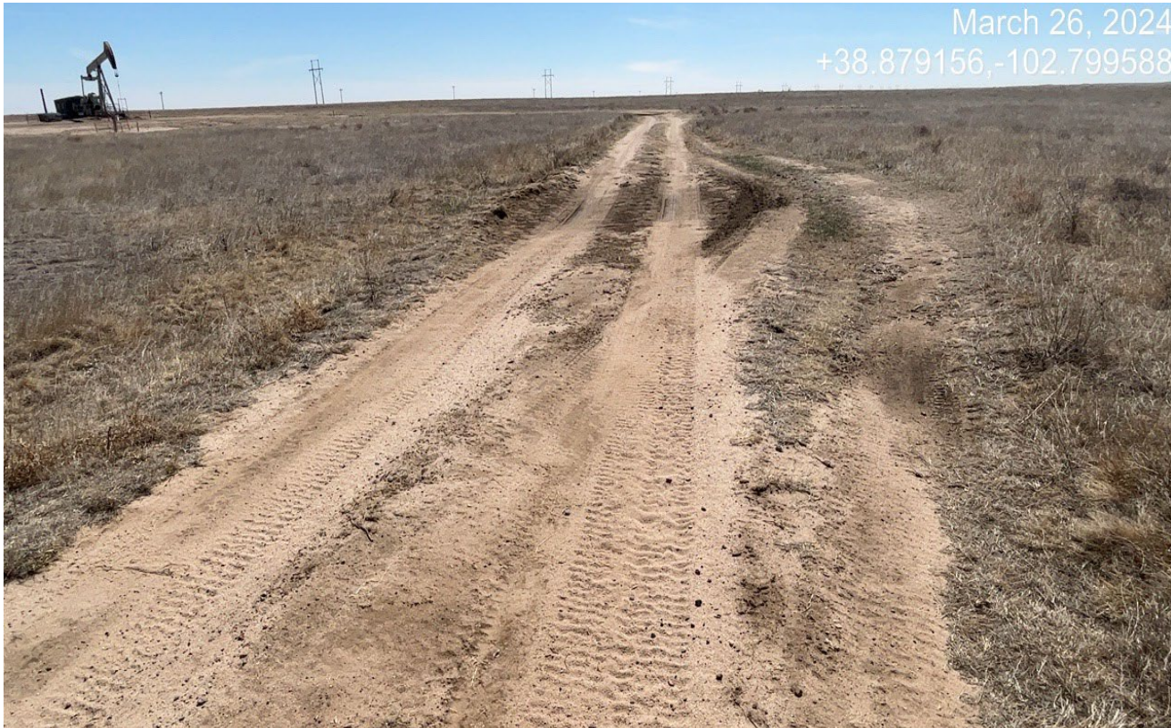
Photo 8. Facing south along the access road. Vehicles are causing unnecessary disturbance driving outside of the access road due to stormwater pooling on the road. The access road must be maintained and shall not drive outside of the access road boundary.
