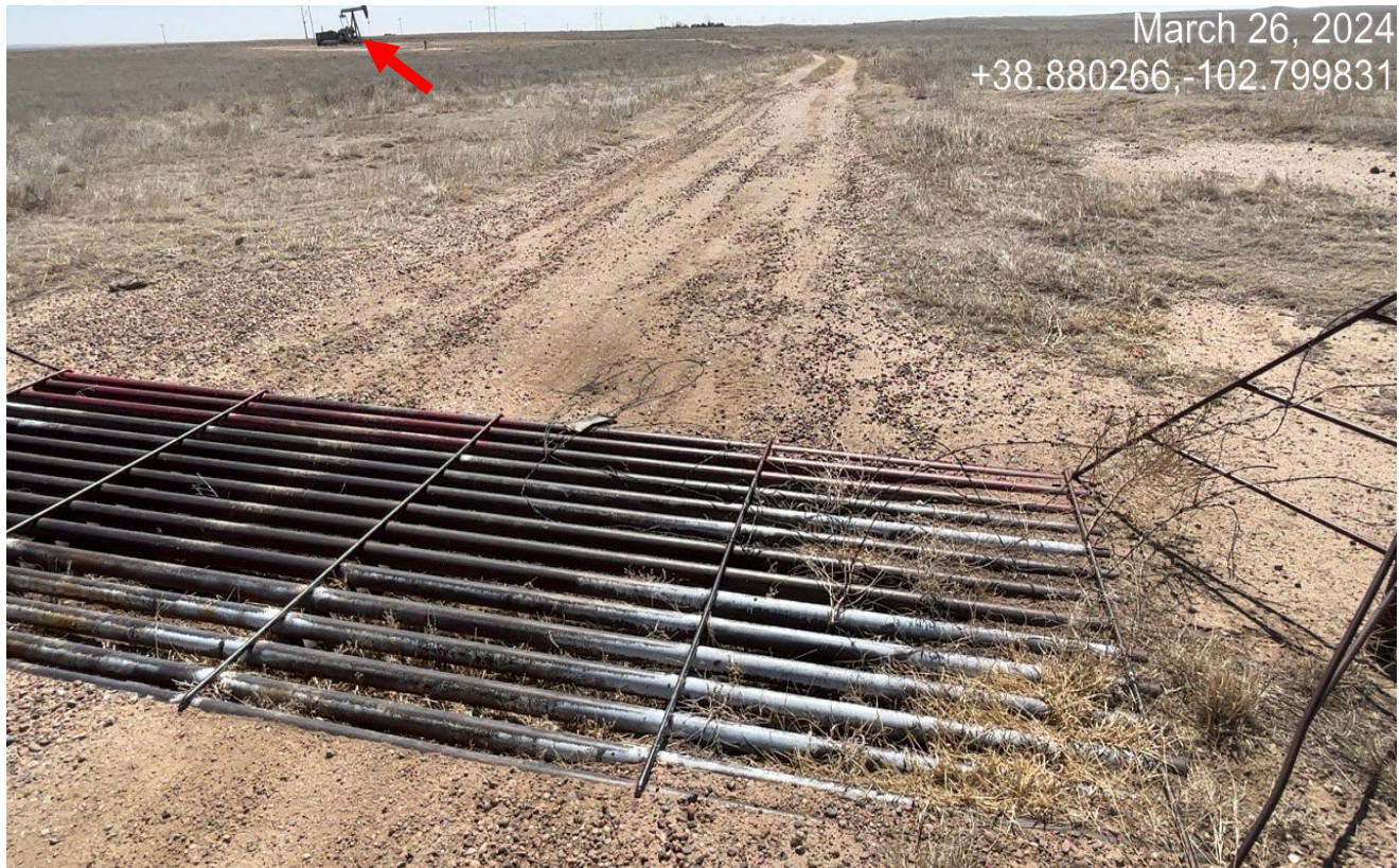
Photo 9. The cattleguard at the beginning of the access road is filled in with sediment and needs to be cleaned out and maintained.
