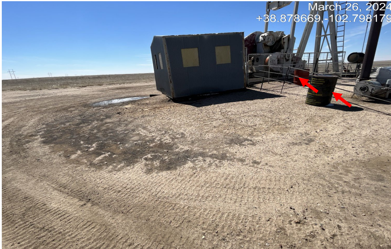
Photo 6. There are chemical barrels with no secondary containment. There are blackened stain soils around the equipment.
