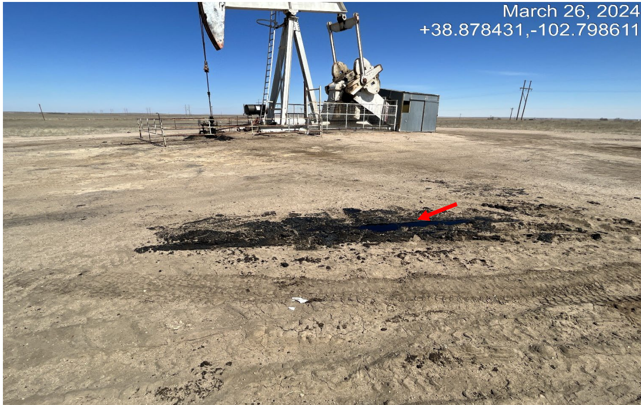
Photo 3. There is oily wasted shown at red arrow that must be cleaned up and properly disposed.
