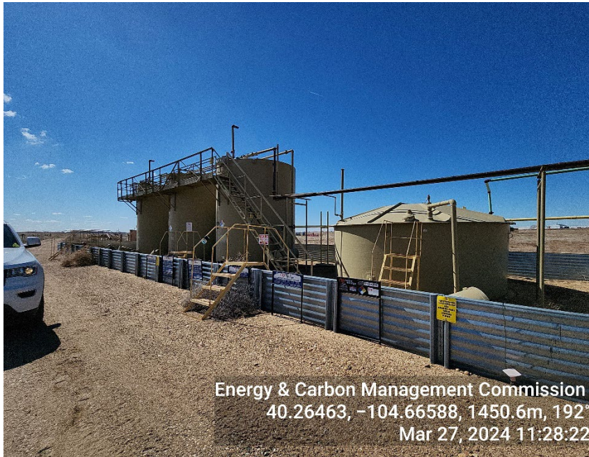
Photo 5: Centralized tank battery
