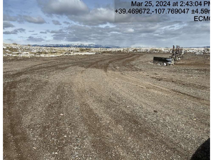
Lack of stabilization/compaction
