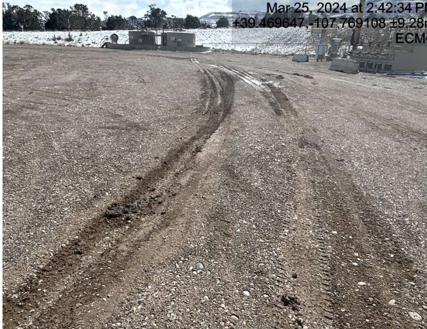
Lack of stabilization/compaction
