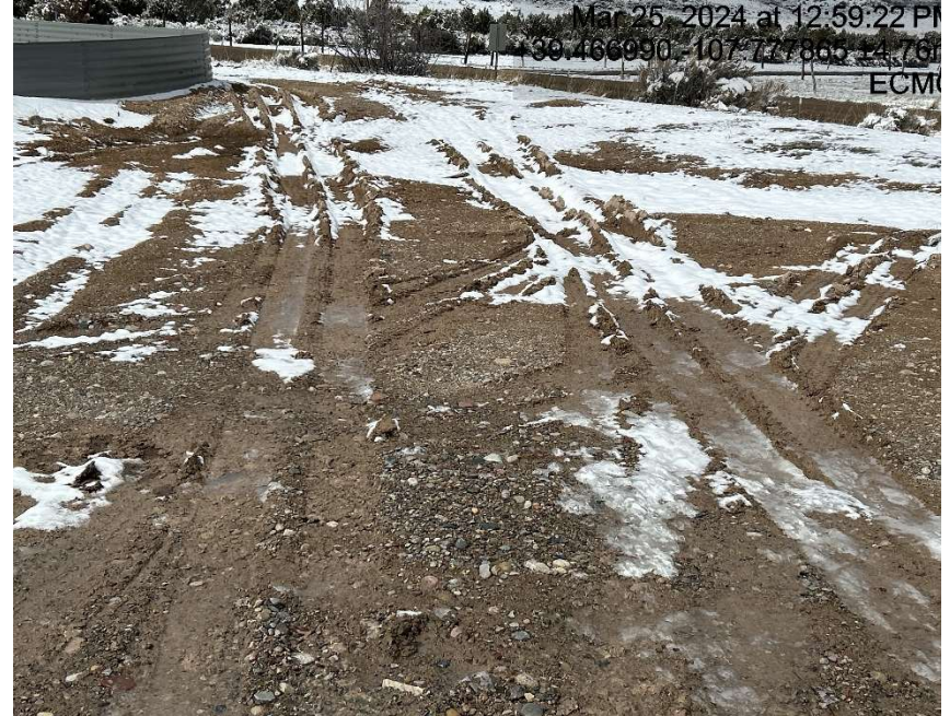
Lack of stabilization/compaction
