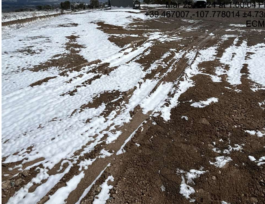
Lack of stabilization/compaction
