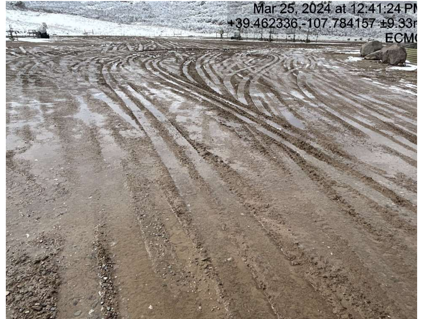
Lack of stabilization/compaction
