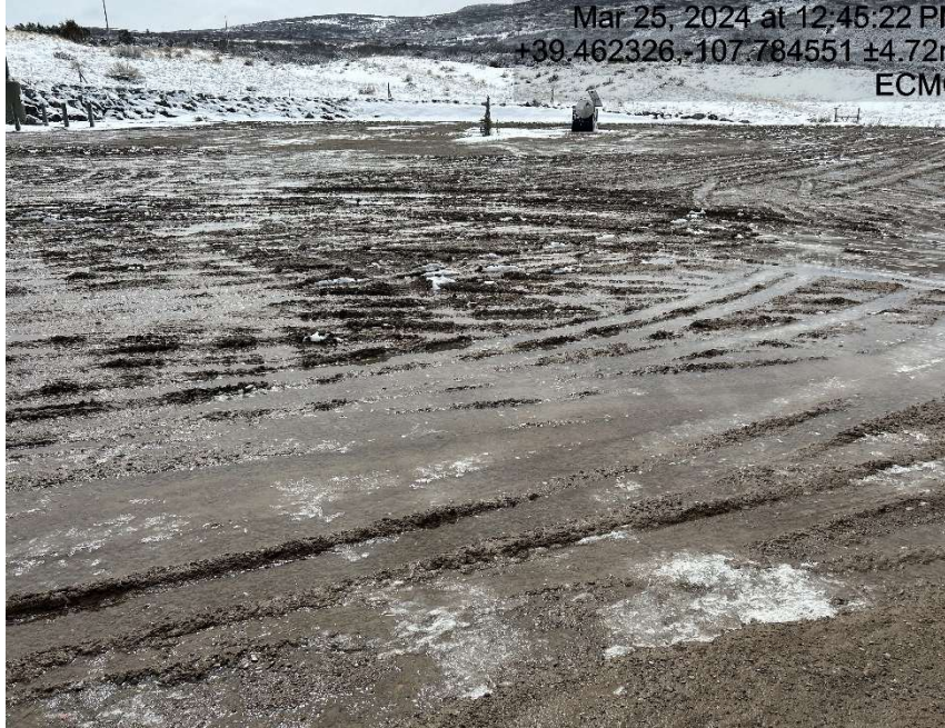
Lack of stabilization/compaction
