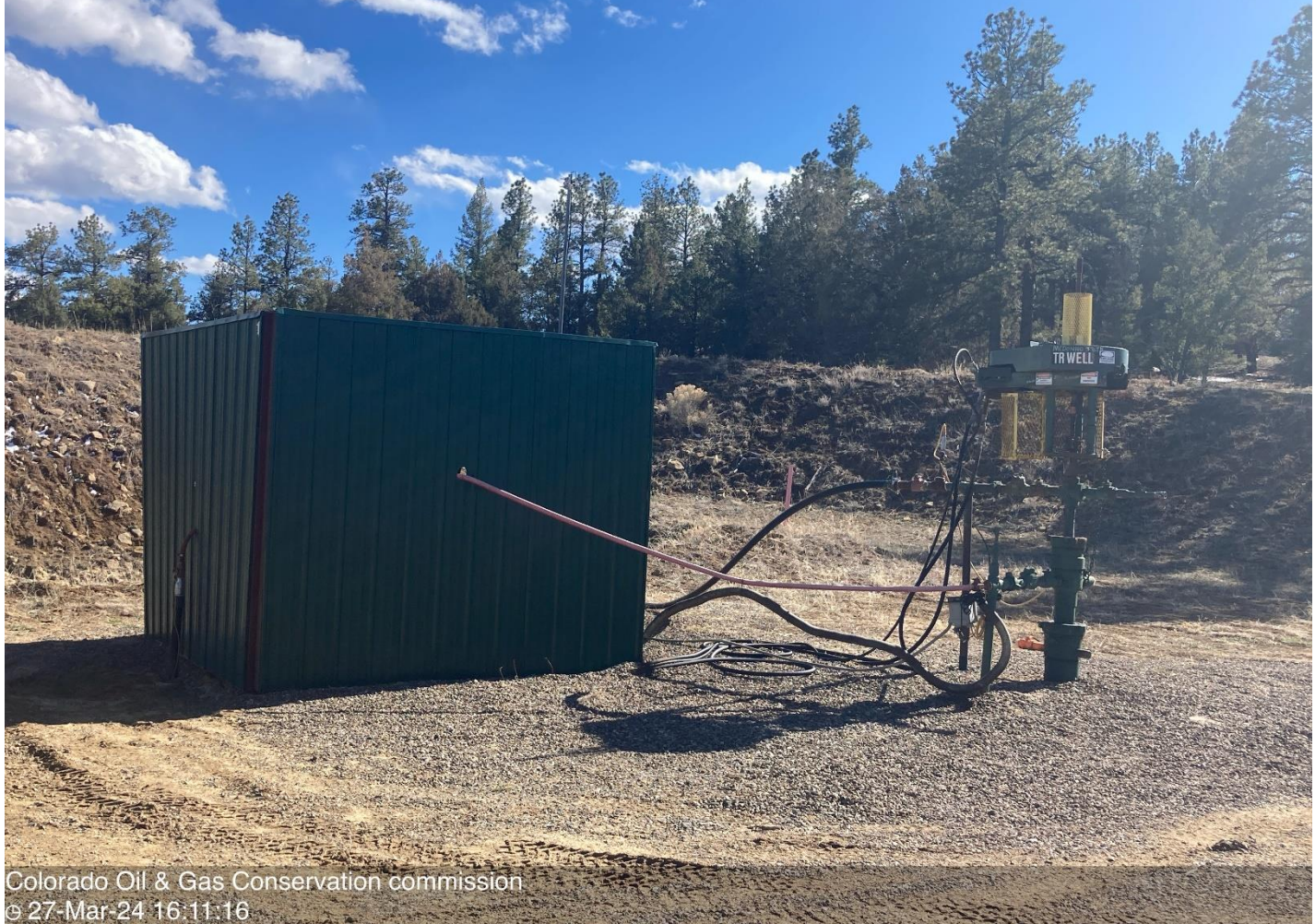
PHOTO 4: TR WELLHEAD AND EQUIPMENT
