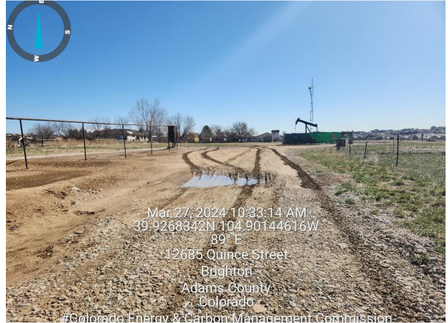
Photo 8 location not draining properly due to improper BMP's
