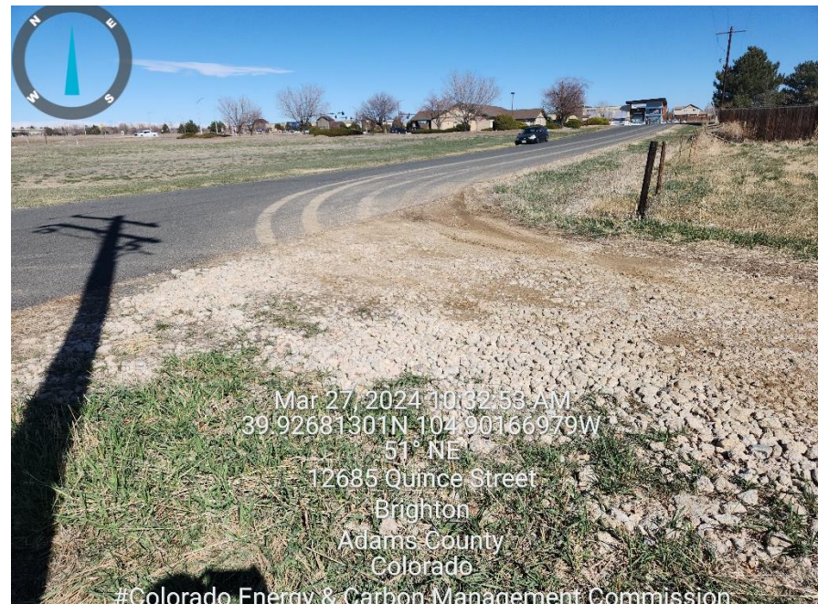
Photo 2 tracking pad in need of maintenance.
