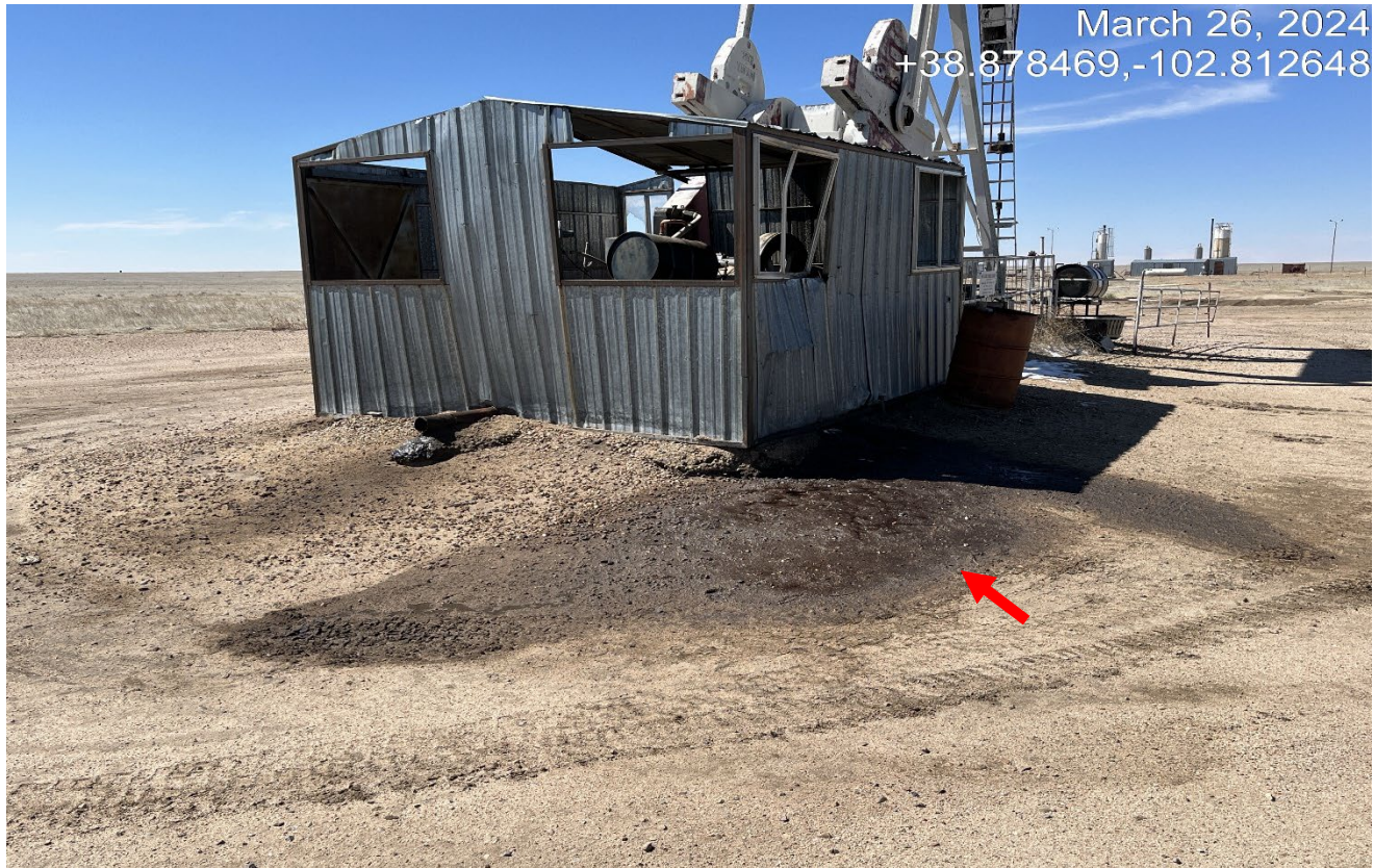
Photo 4. Facing southwest toward the engine compressor. There is oil saturated soils that have leaked out of the engine compressor. The leak must be controlled and impacted soils removed.
