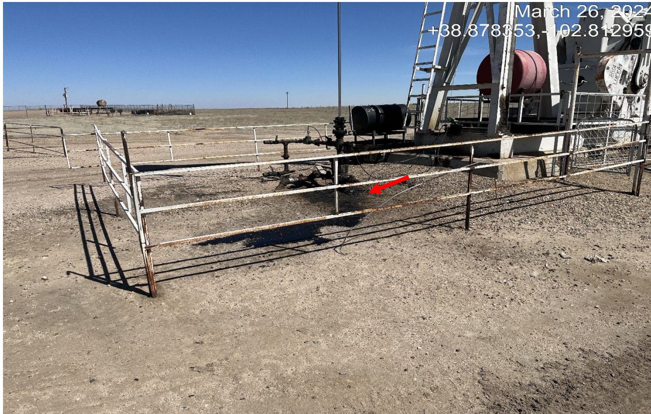
Photo 2. There is oil leaking out of the wellhead that must be controlled and cleaned up.
