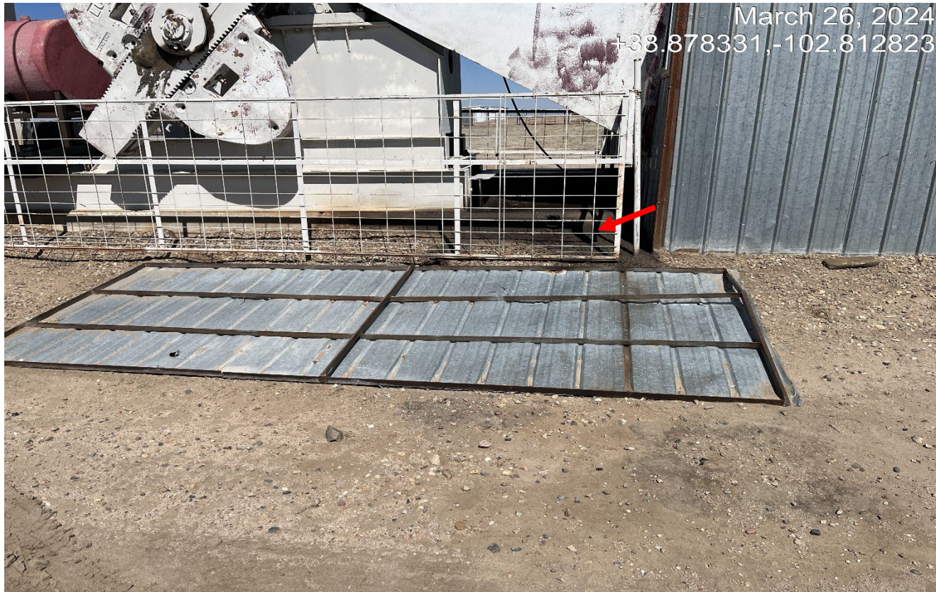
Photo 3. There is a panel laying on the ground that needs to be removed. There is oily fluids leaking out of the pumpjack at red arrow.
