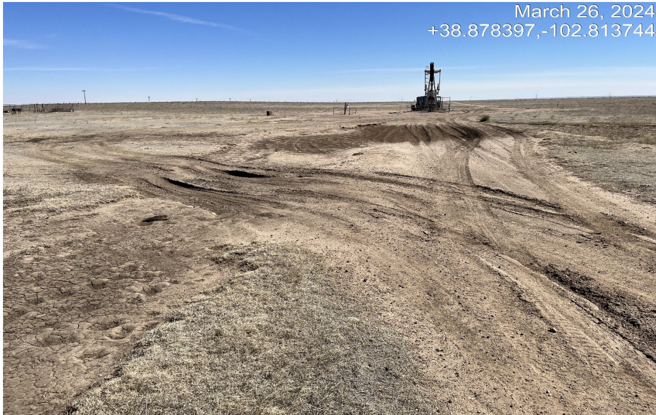
Photo 1. Facing east along the access road. Vehicles are causing unnecessary disturbance driving outside of the access road due to stormwater pooling on the road. The access road must be maintained and shall not drive outside of the access road boundary.
