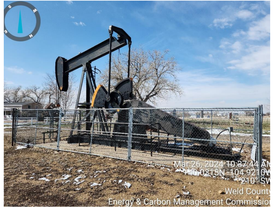
Photo 2 well head and equipment
