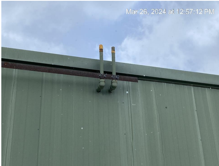
Relief riser missing rain protection
