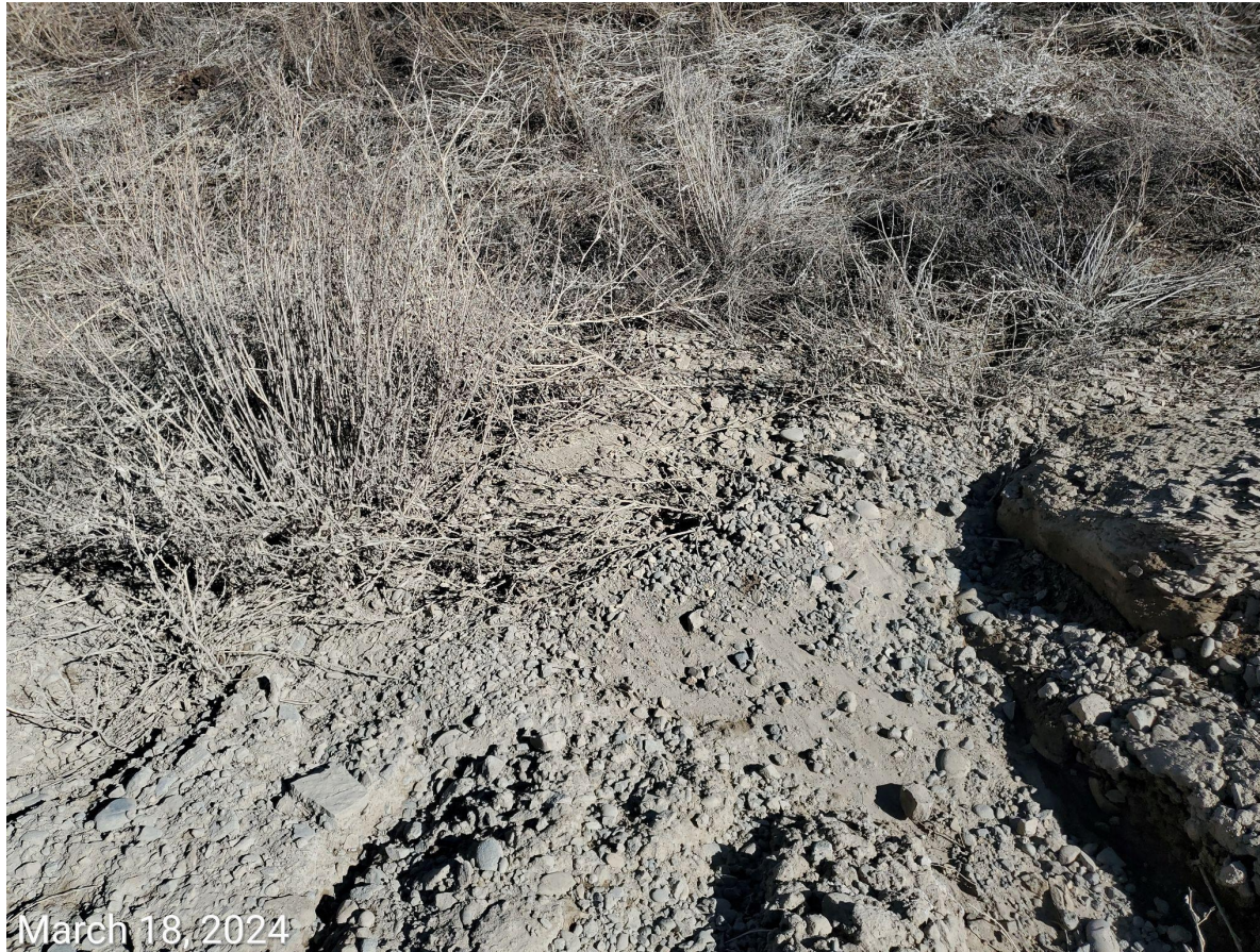
Photo 10: Sediment transport and deposition due to runoff and erosion degradation at the access road.
