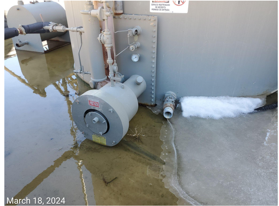
Photo 5: Photos examples showing lines at tanks missing required cap/plug.
