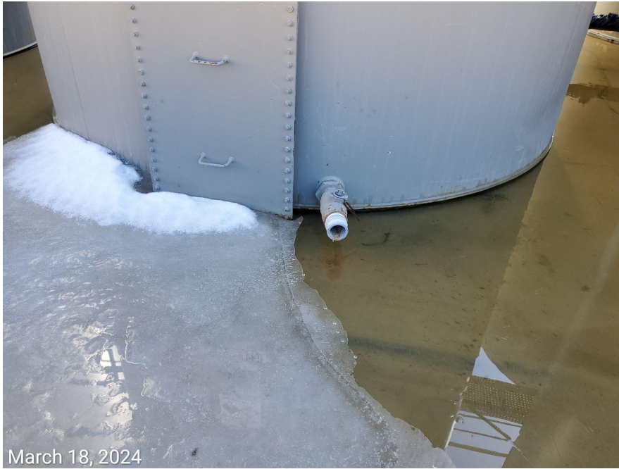
Photo 5: Photos examples showing lines at tanks missing required cap/plug.
