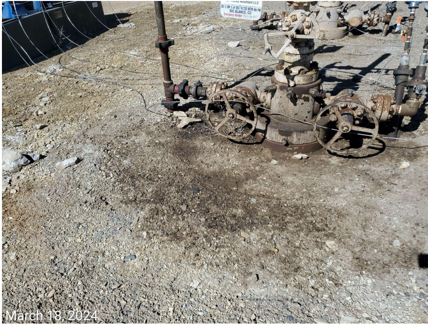
Photo 7: Photos example showing stained soils remaining around the wells.
