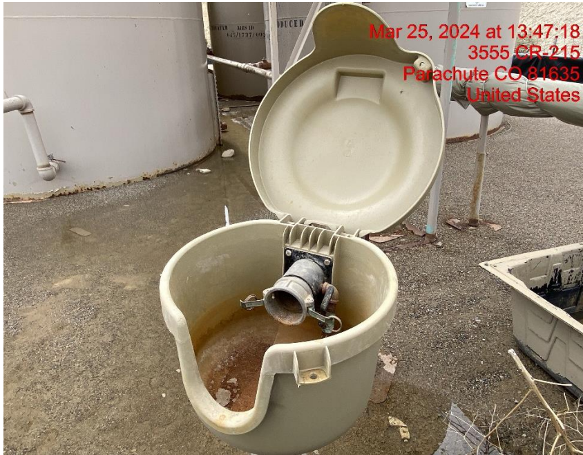
Open-Ended Load Line – Photo #00076
