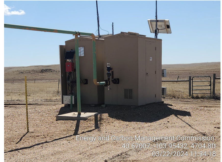
Photo 10 – Gas Meter Houses
