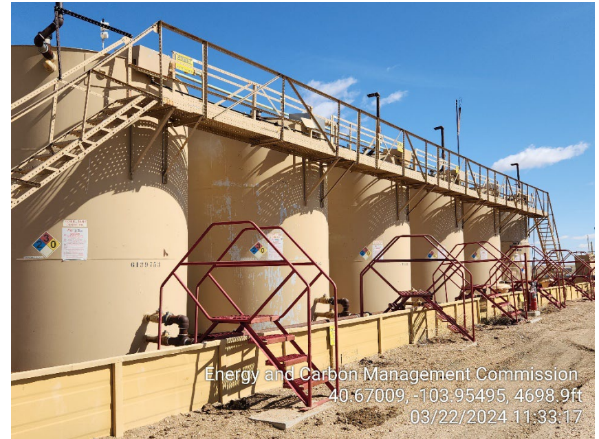
Photo 6 – Tank Battery
